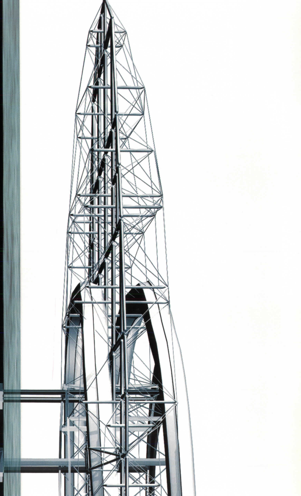
View of tensegrity structure
