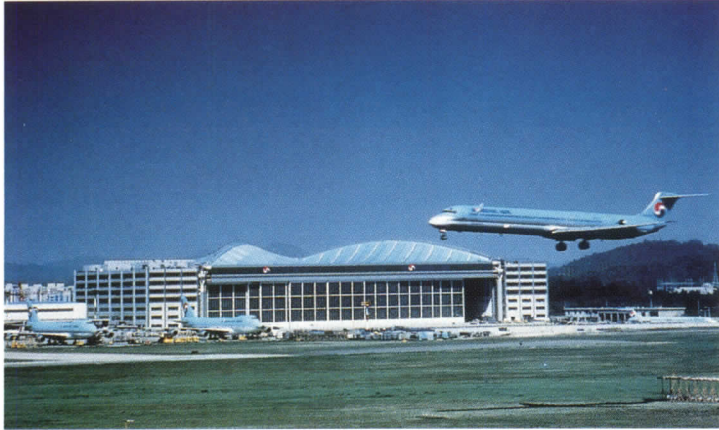
The new Korean Airlines headquarters in Seoul (above) brings maintenance and management together. The roof truss (facing page, bottom) was assembled on the ground and then hoisted to the roof. The double top chord (facing page, top) of the bow arch straddles the supporting box columns.
