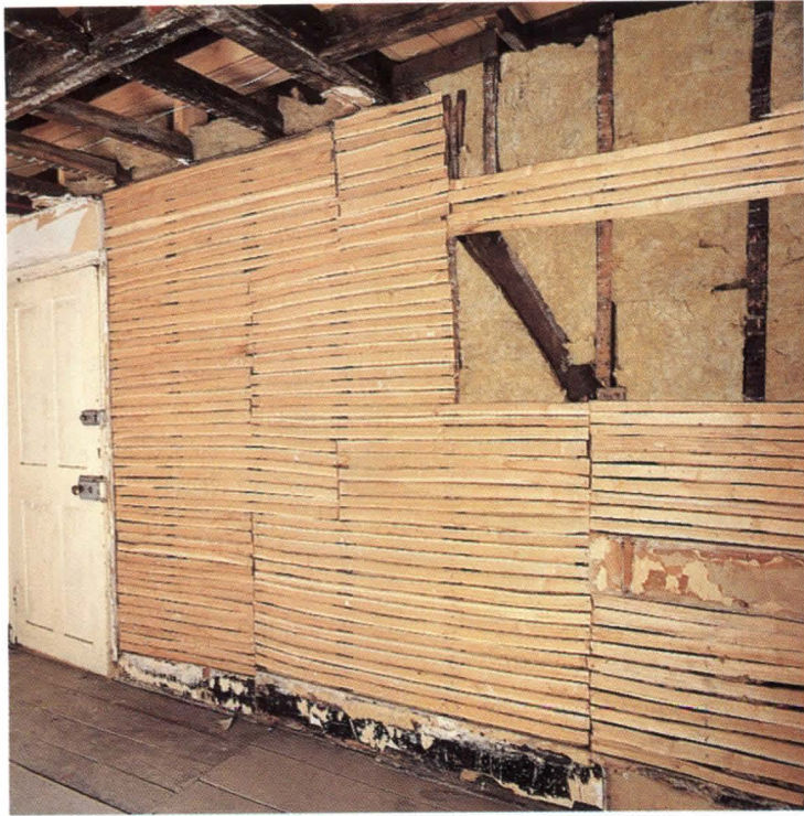
Insulation was installed behind new hand-stripped chestnut laths in top-floor bedroom.
