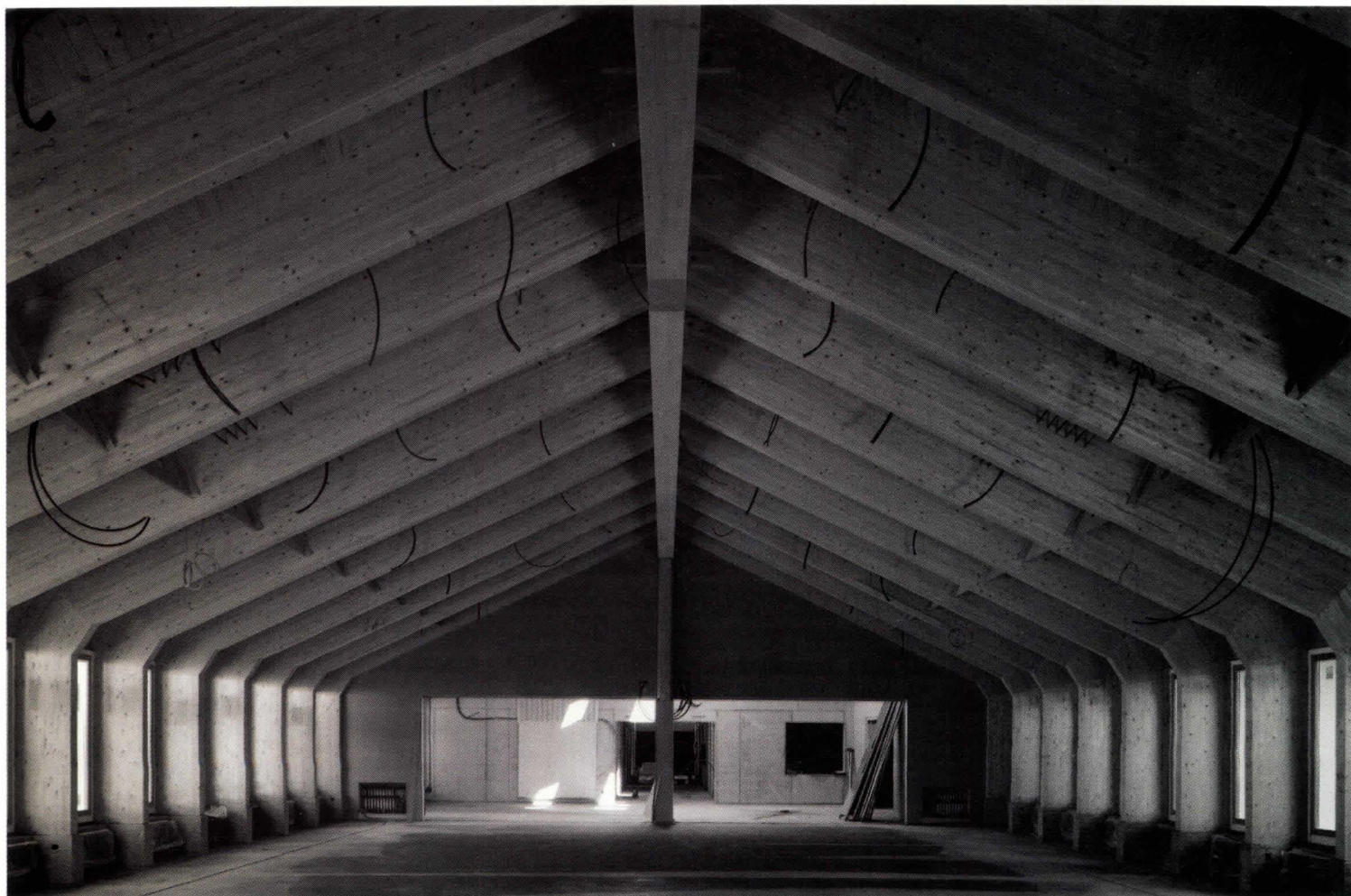
Interior during construction
