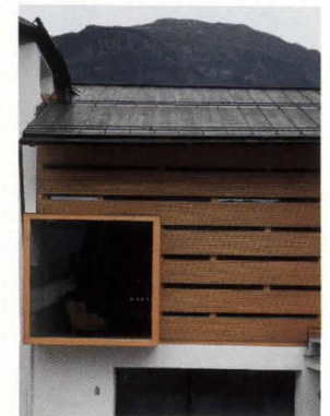
Detail at bay window
