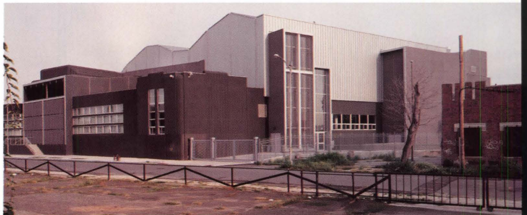
Views of church (from top to bottom) punctuate barren, light-industrial character of its Queens, New York, neighborhood: Oblique view of north and west facades shows church at its most formally expressive; ground level drops 12 feet behind low white wall bounding parking lot. On west facade, glazed rectangular volumes, or "tubes," mark principal entrances to church; translucent fiberglass panels clad subsidiary corridors at back of sanctuary. On south facade, one tube curves to screen approximate center of art moderne original. Vertical glazed projections along west facade mark reciprocal, secondary entrances to "tube" corridors.
