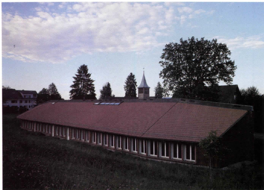
Exterior showing fish-scale shingle roof
