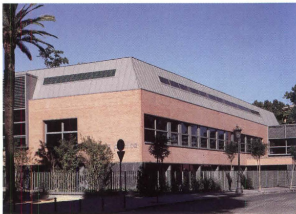
On more exposed west elevation (top), louvered screens help diffuse intensity of Sevillian. Library's long, low volumes are capped by zinc mansard roof (above) with clerestories that bring light into book-stack areas. Stacks are arranged around perimeter of library, overlooking double-height reading room (facing page, top). Luminous reading area connects with secluded patio at heart of library (facing page, bottom right).
