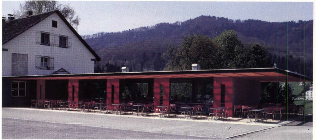
Addition and existing building
