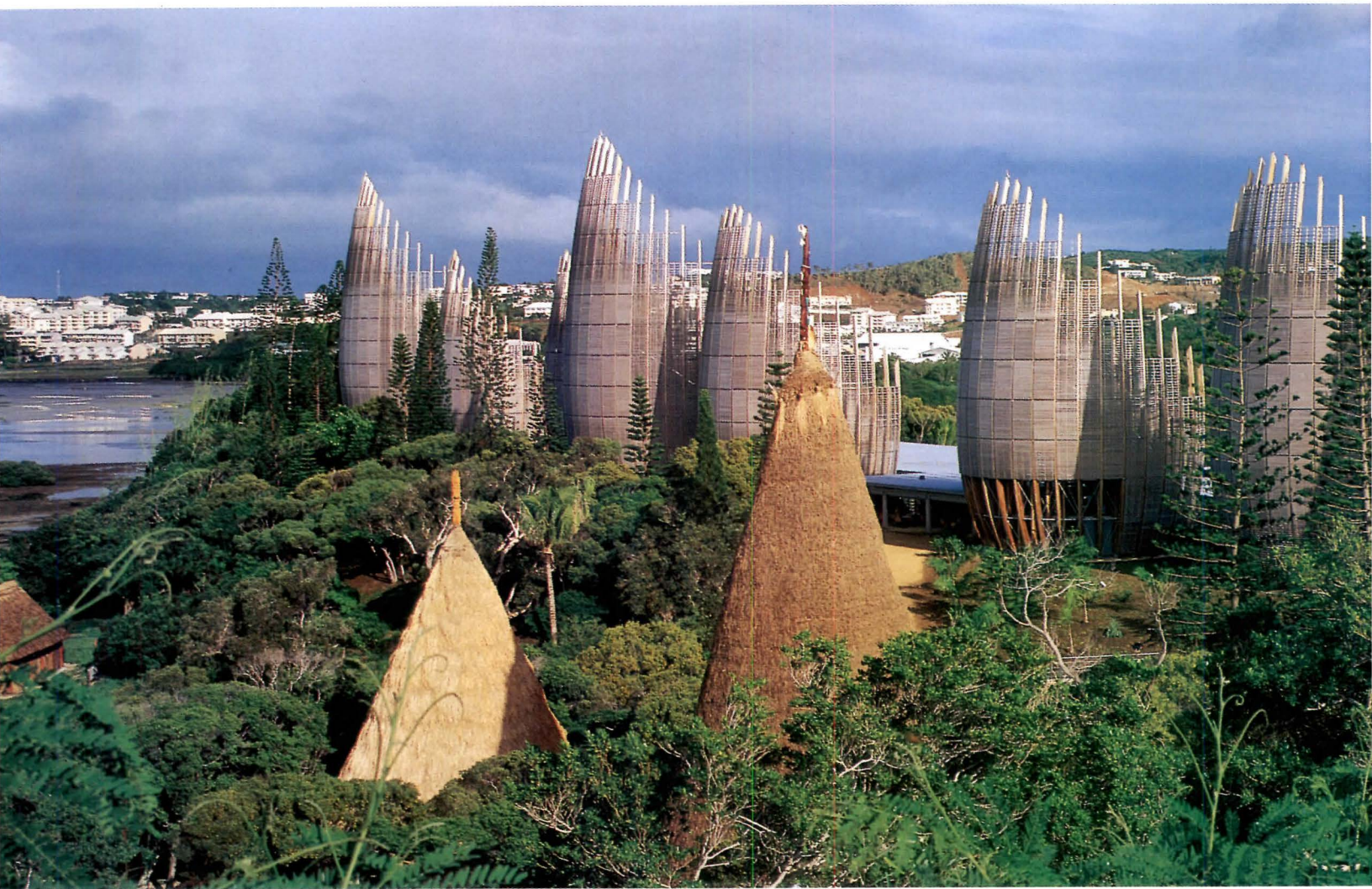
Wood cases of Tjibaou Cultural Center (previous pages) bow out toward bay; their glue-laminated ribs rise over flat-roofed structure and surrounding gardens and lagoon.
