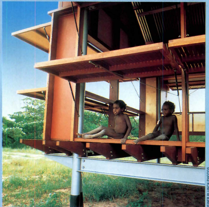
Simpson-Lee House (1994, top) and Marika-Alderton House (1994, above) demonstrate Murcutt's concern for climatic and cultural context through use of vernacular forms, simple materials, shading devices, and natural ventilation.
