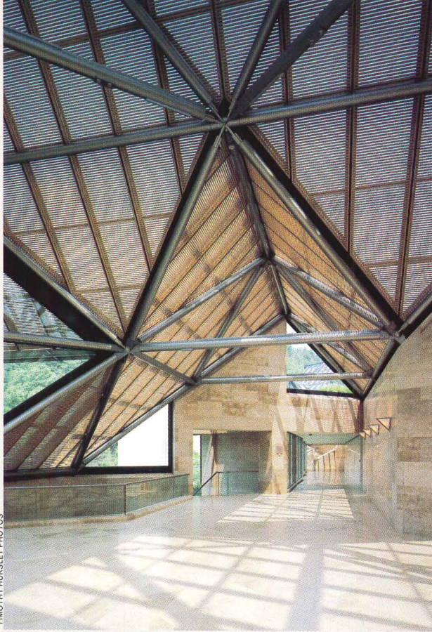
In north corridor (left), horizontal steel members of tetrahedron conceal emergency lighting and uplighting. Typical 19-centimeter-diameter cast-steel node (below) is positioned on center line of module. Wall position is represented by darker line at left.
