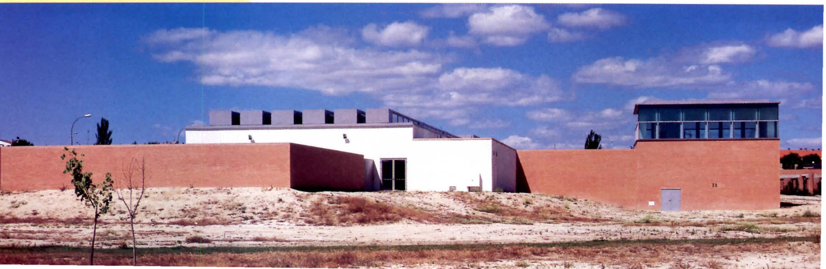
East facade is framed by brick-enclosed patio (left) and library (right).
