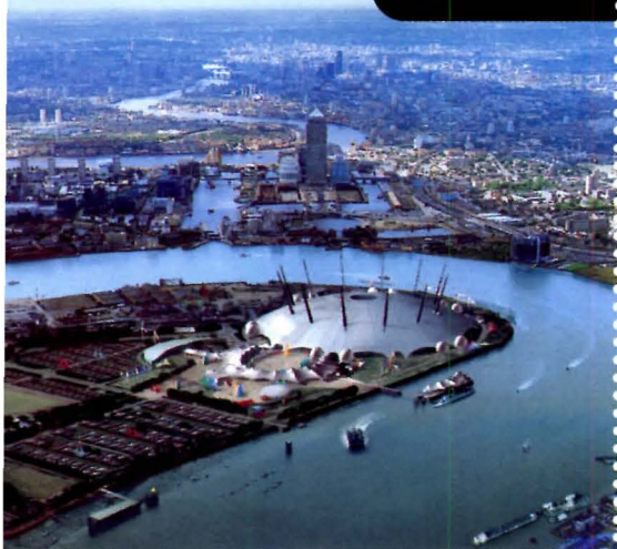
Tensile dome by Richard Rogers (above) covers site in Greenwich. Michael Wilford & Partners' Lowry Center in Salford (bottom) exemplifies lottery funding success.
