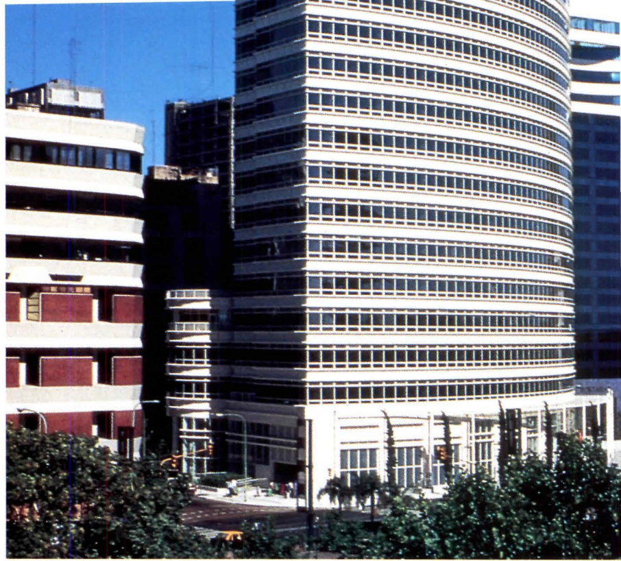
In designing 21-story office building in Buenos Aires, Cesar Pelli & Associates worked within city's restrictive construction code, which limited building's massing to 35 percent of site.
