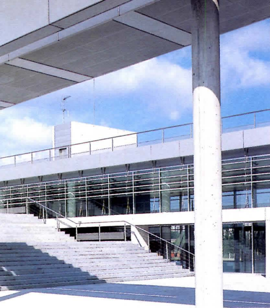
Monumental granite staircase ascending from river bank slices through entry block in bold, urban-scaled gesture. Concrete colonnade frames entry plaza and stair.
