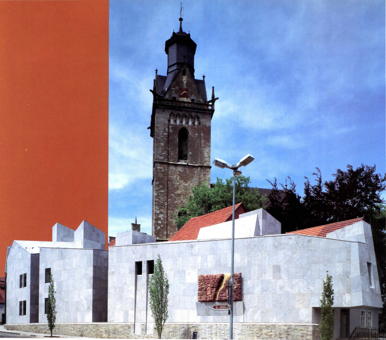
Bavarian limestone-clad galleries wrap southern edge of site along Stechbahn (above).
