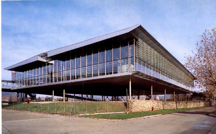
Block containing permanent exhibition galleries hovers over ruins of Roman-era house on metal pilotis . Elegant, fritted glass-clad brises-soleil are tensioned between delicate steel cables to shade interiors.
