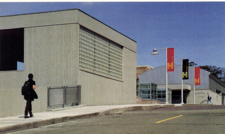
From campus, entrance to addition and courtyard is marked by flags. Concrete structure (foreground) houses stairs and elevator to garage. Vaulted roof encloses entrance and theater.
