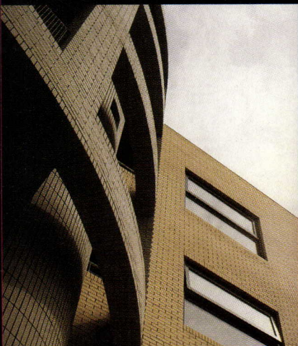
Thin-layered masonry faces mixed-use complex in Hoorn, the Netherlands.
