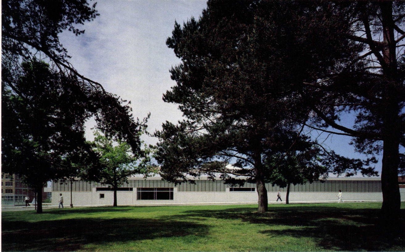
Offices, theater, classrooms, and support spaces occupy bar building to east of original Henry gallery. Large window (at center) illuminates main staircase to new galleries.
