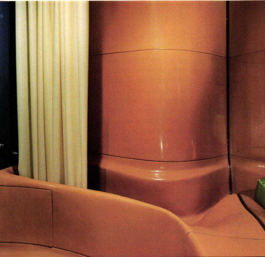
Molded fiberglass bathtub (left) and shower stall (right) were fabricated in sections small enough for the building's freight elevator. Hinged panels permit service access to pipes and plumbing fixtures.
