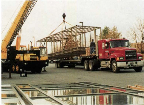
ABOVE LEFT: Student design/build team specified low-e glass to increase energy efficiency of Nomadic Transit Module, to be completed next year. ABOVE RIGHT: Students completed computer models of modular structure before construction began. FAR LEFT: Steel house and adjacent Battery Barn are located outside CUA architecture school. LEFT: Steel frame was lifted by crane and transported by truck.
