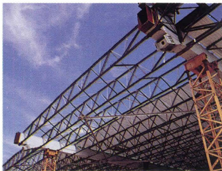
90' Vulcraft steel joists.
