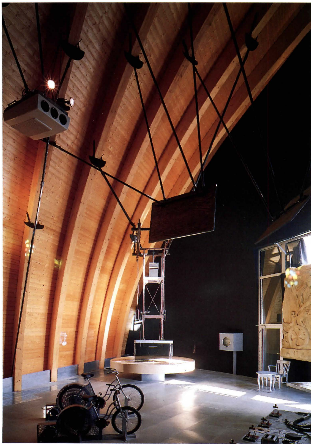
FACING PAGE: Sloped window projects from zinc-clad exhibition hall. Small lake separates building from road. ABOVE: Exhibition hall is framed in laminated timber beams and features displays of energy generation and distribution principles designed by Craig Hodgetts and Ming Fung.
