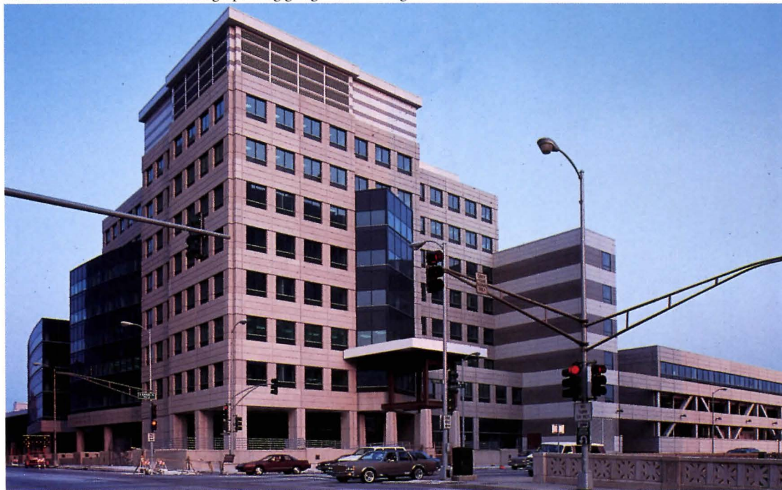
CORNER VIEW: Clumsy assemblage of precast, glass, and steel proves that less is more.
