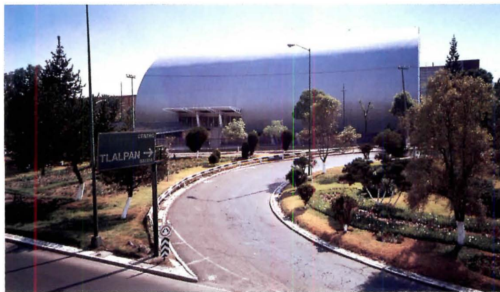
ABOVE: National School of Theater, on the campus of the City of the Arts in Mexico City, includes a theater, library, and classrooms. THESE PAGES: Steel-truss-supported steel canopy (right) pierces shell, forming the theater's main entrance.
