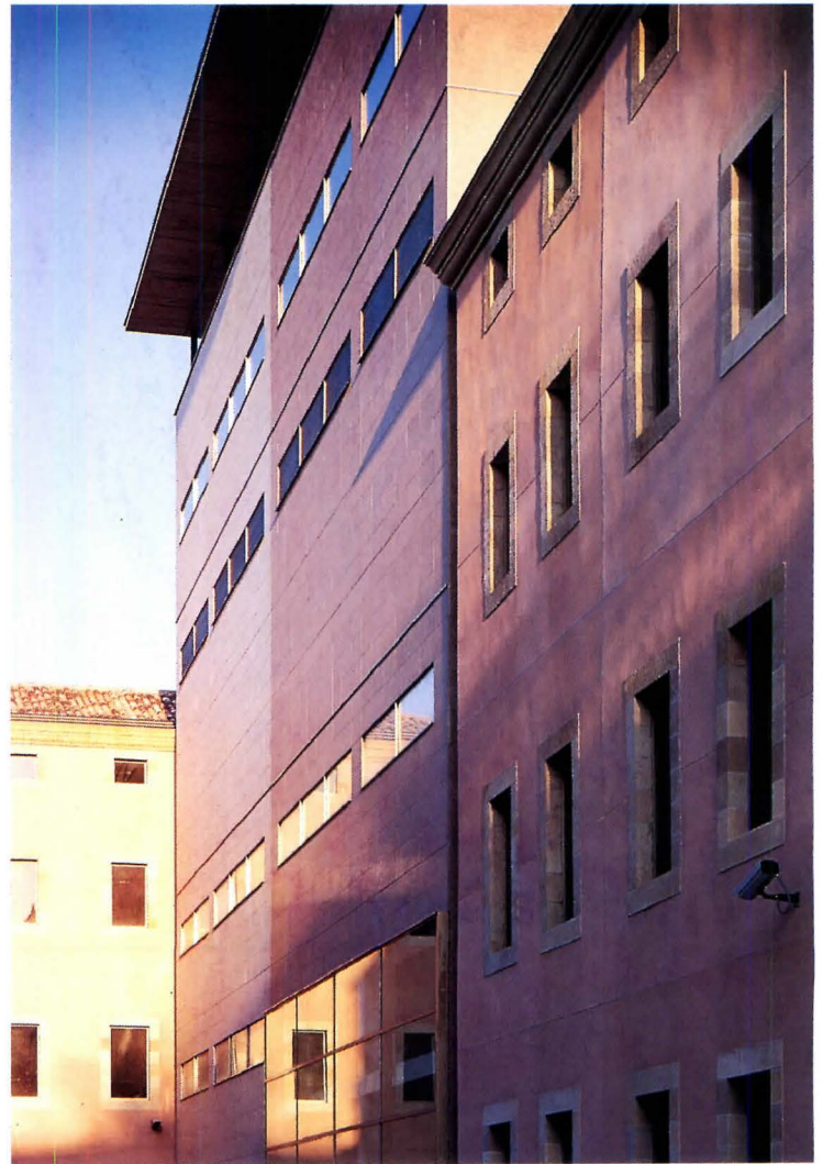
ABOVE: Viaplana and Piñón clad rear facade of new cultural center in granite (left) to harmonize with stucco of 1802 charity hospital (right). FACING PAGE: Courtyard facade of new entry hall is clad in double-paned thermal glass in two shades of gray.
