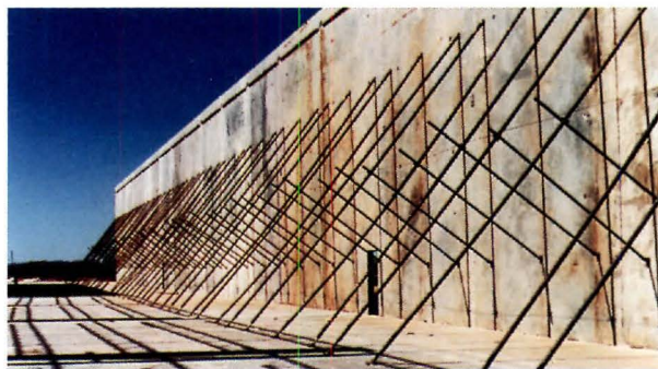
ABOVE: Steel chord angles fastened to wall panels support metal roof.
