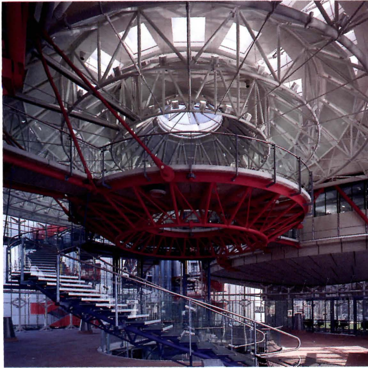
ENTRANCE HALL: Helical staircase incorporates vestibule to courtrooms.
