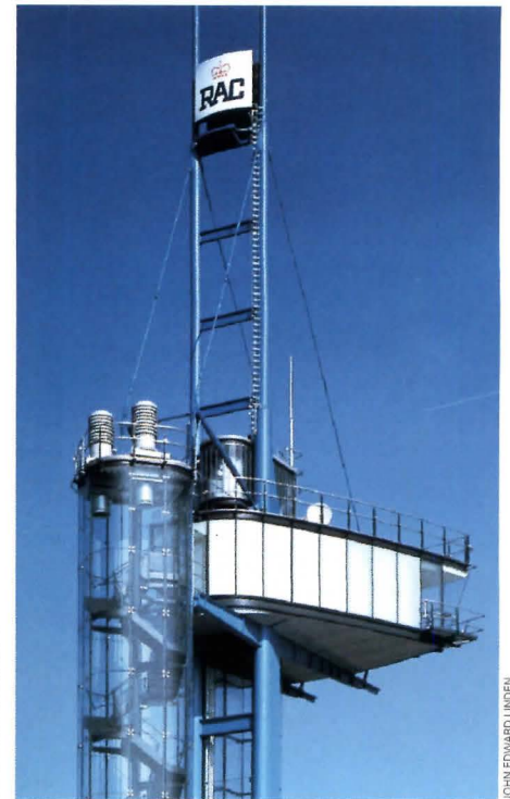
SPIRE: Glazed elevator leads to visitors' room.
