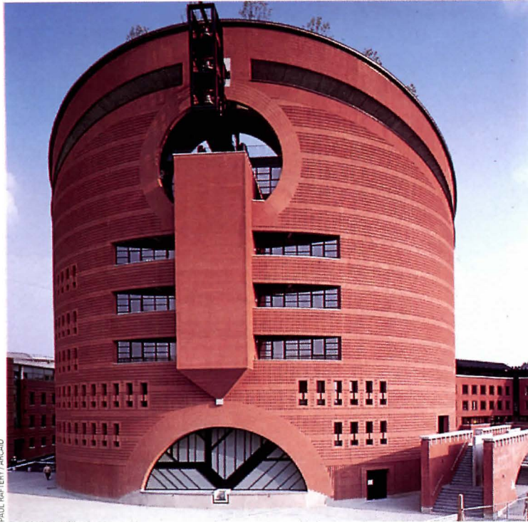
CYLINDER: Brick-enclosed stair leading to belfry projects from main volume.
