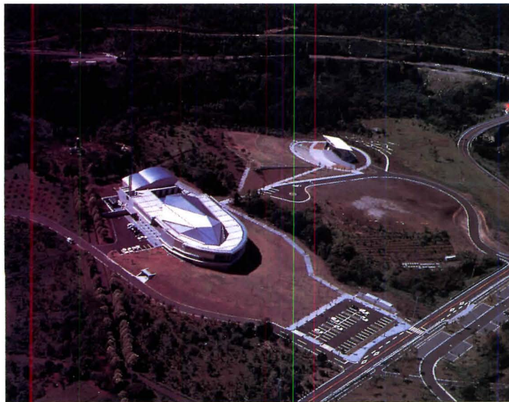
ABOVE: Located on Kyushu Island, Kirishima International Concert Hall comprises main auditorium (left) and outdoor theater (right). THESE PAGES: Foyer and bar are visible through east end. Roof is clad in 0.4 millimeter-thick stainless steel.
