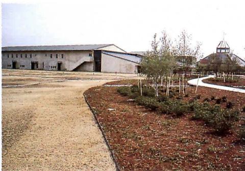
TOP: Rock salt was added to concrete walls to create texture. CENTER: Bays of classroom building are topped with precast concrete roof. ABOVE: Tilt-up construction minimized building costs of religious campus. DETAIL, TOP RIGHT: Tilt-up panels are joined with steel-headed studs. DETAIL, CENTER RIGHT: Steel plate supports beam seat for wood floor joist. DETAIL, RIGHT: Tilt-up wall supports wood joist (right) and concrete roof.
