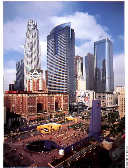
BAD PARK: Renovated Pershing Square in Los Angeles.
