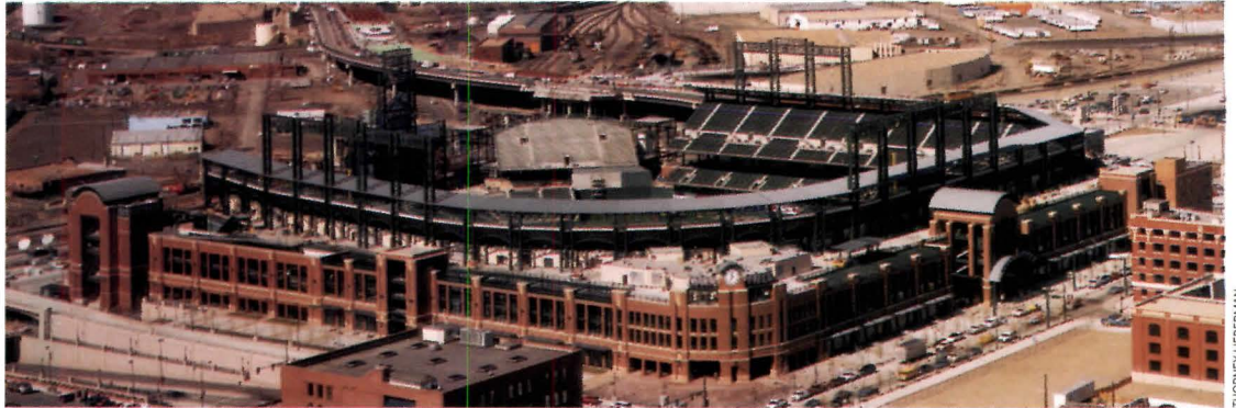
AERIAL VIEW: Coors Field's brick and sandstone facade and steel superstructure reflect industrial setting in Denver.
