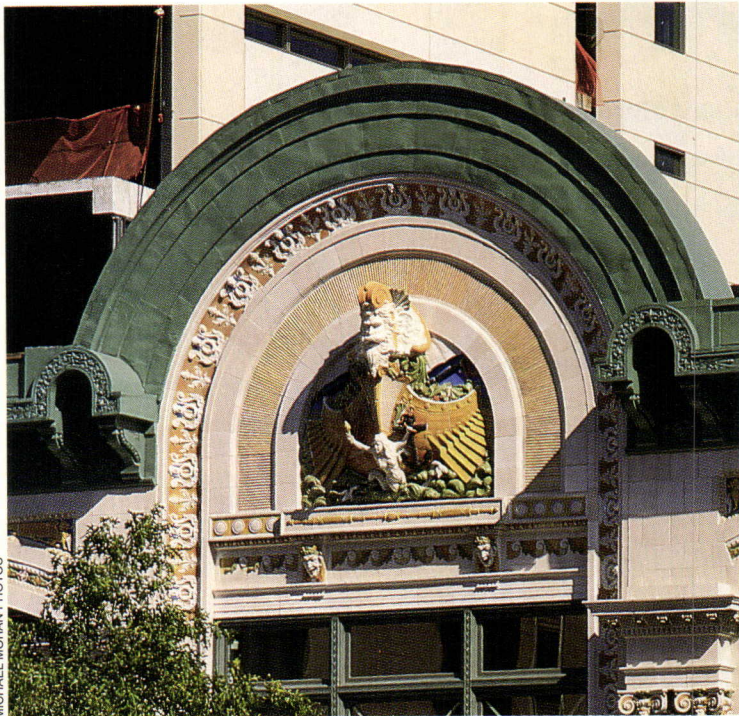
ENTRY DETAIL: Ornament restored with new and salvaged terra-cotta.
