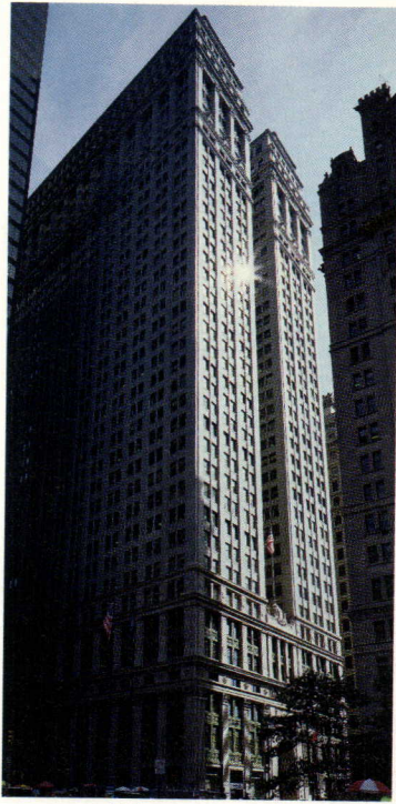
EQUITABLE: Masonry repaired.
