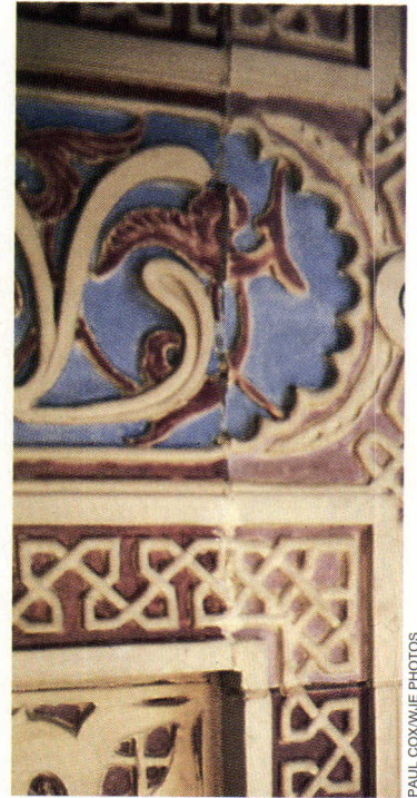
TRACERY DETAIL: Glaze colors restored.
