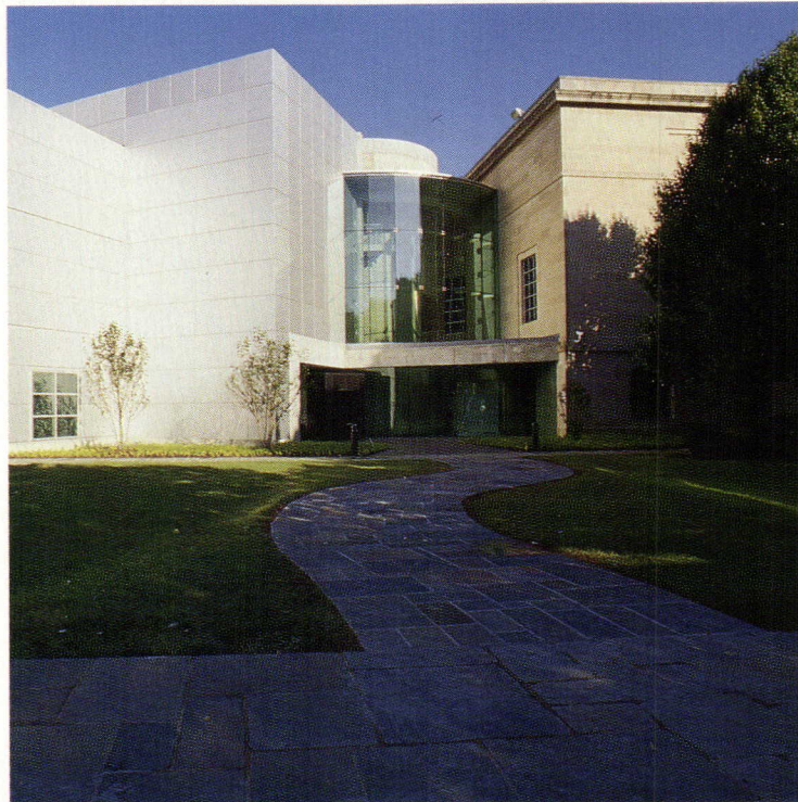
NEW MEETS OLD: Addition is linked to original by glass and concrete rotunda.
