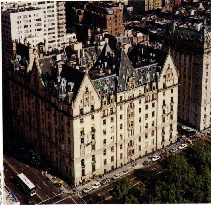
DAKOTA EXTERIOR: Repair quantities determined by surveys from a distance.
