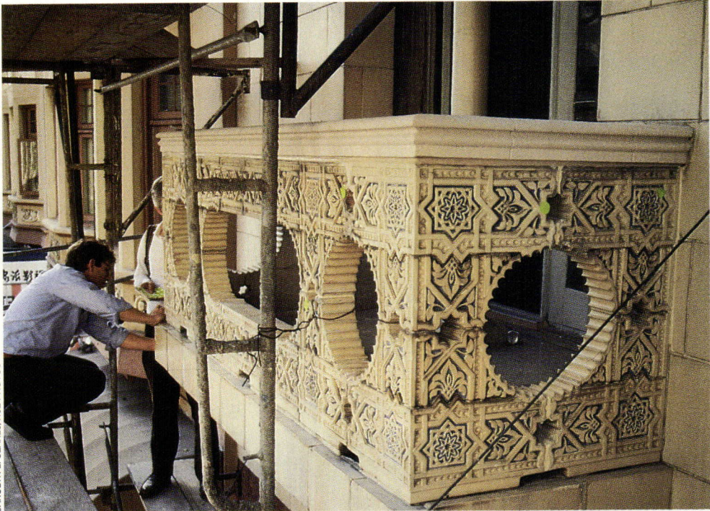
BALCONY RAILING: Terra-cotta restored and seismically strengthened.
