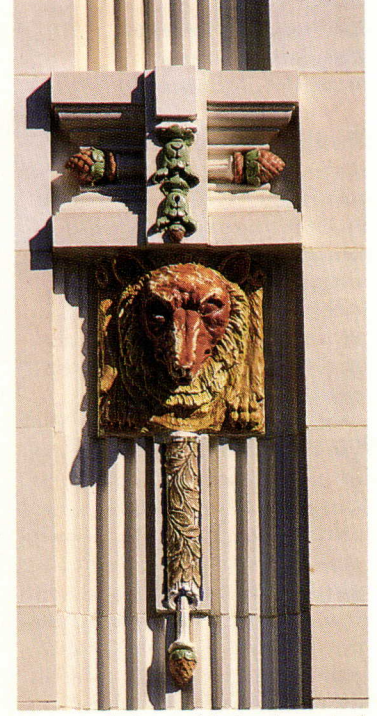
DETAIL: Polychromed foxheads repaired.
