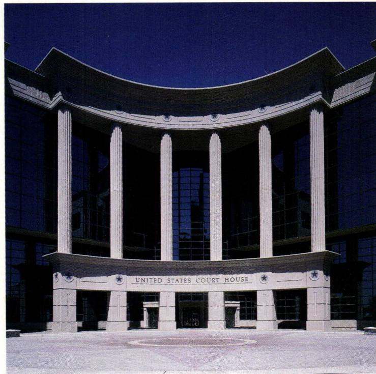
SHREVEPORT COURTHOUSE: Fast-track project required accelerated reviews by GSA.
