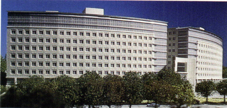
IRS HEADQUARTERS: Educated guesswork was required to fit systems into structure.
