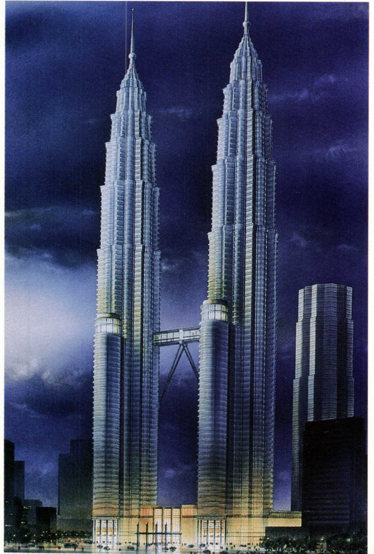
TOP: SOM/Chicago's Plaza Rakyat, in Kuala Lumpur, provides urban open space shaded from equatorial sun.
