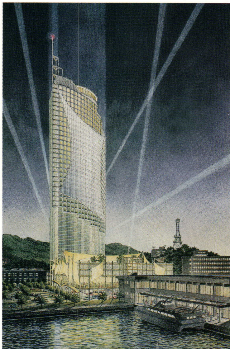
TOP: Jeffrey M. Kalban & Associates' Tianjin Times Square complex incorporates curtain wall except where concrete frame required punched windows. ABOVE: The Shekou Harbor Building, by Loeb Schlossman & Hackl in Shenzhen, required 48 approvals.
