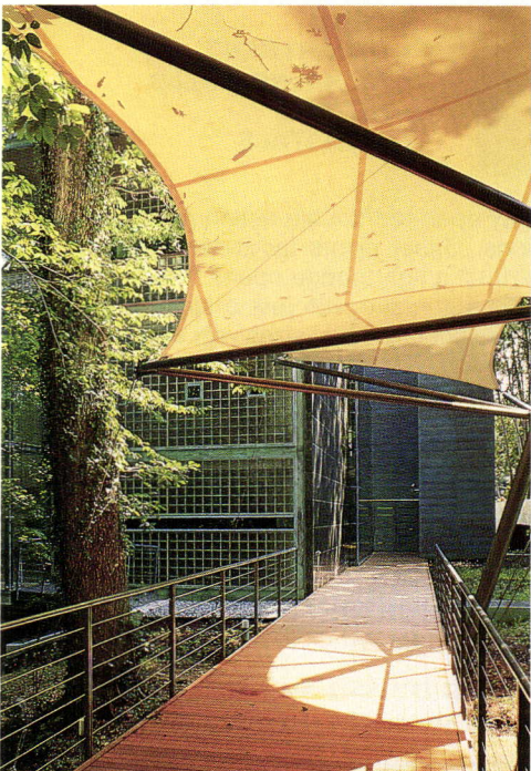
FABRIC-COVERED WALKWAY: Spans Rock Creek Park.
