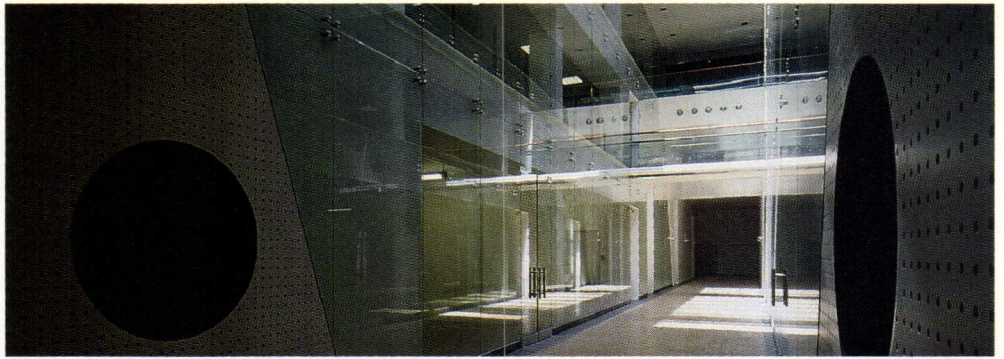
UNDERGROUND LABS: Atrium is topped by glazed roof and enclosed by laminated-glass partitions.
