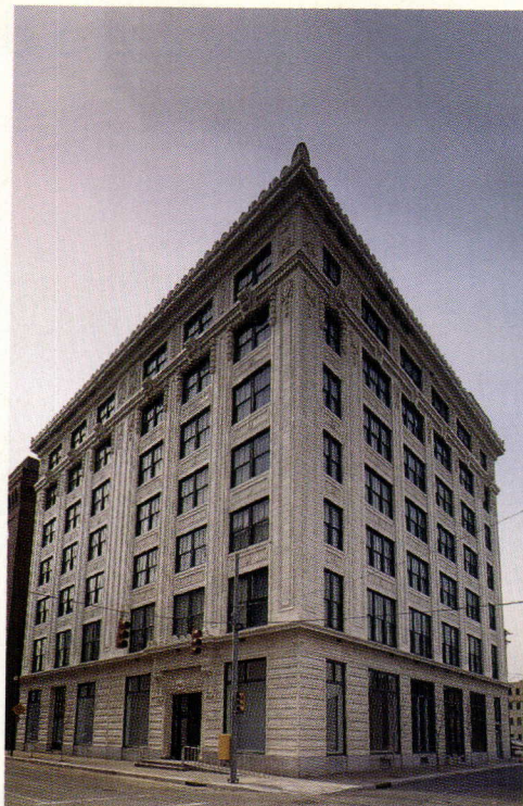
WARHOL MUSEUM: Terra-cotta facades are restored.
