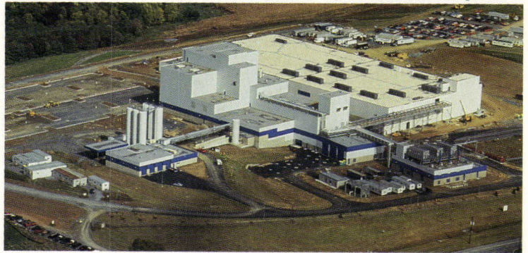
AERIAL VIEW: Final form of building resulted from processing sequence.
