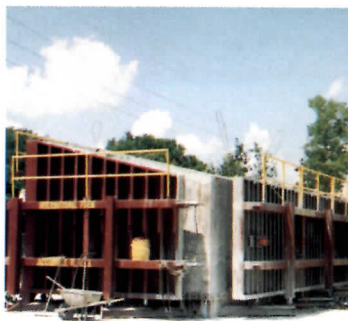
FORMING MACHINE: Jackets secure concrete.
