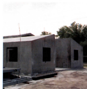
SHELL: Finished in 48 hours.
