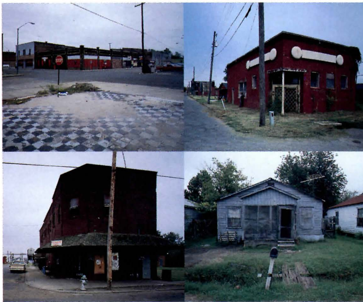
HAT members proposed new middle- and low-income housing to occupy vacant blocks in downtown Helena (top left). Despite the deterioration of retail buildings (top right and bottom left) and existing housing (bottom right), the small Arkansas agricultural town retains much of its community fabric. In addition to a new residential zone, the HAT plan calls for an expansion to Helena's commercial district.
