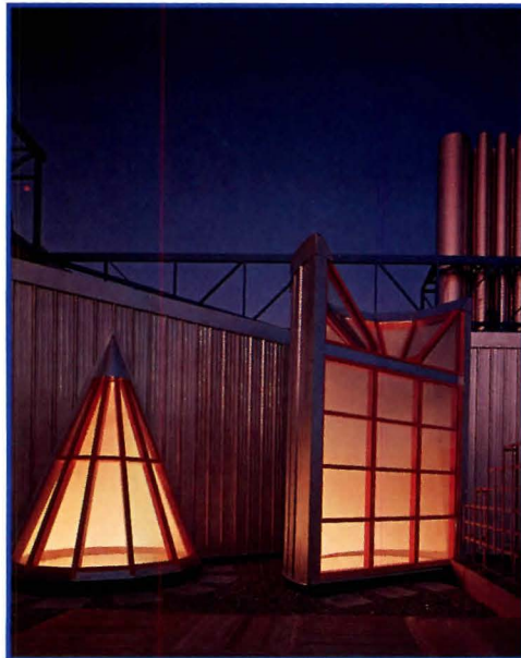
New addition's corrugated, metal-clad facade (right in facing page photo) contrasts with open concrete frame of 1977 Wellesley College Science Center (below). Interior spiral staircases are daylit through sculptural roof monitors (above).
