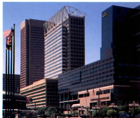
SOM tower is inserted between Belluschi's 10-story building (top drawing, left), and new parking garage (second and third drawings). Bay is supported by trusses (fourth drawing). Window rhythm reflects 1974 building (facing page, inset), while shaft harmonizes with neighboring towers (above and right).
