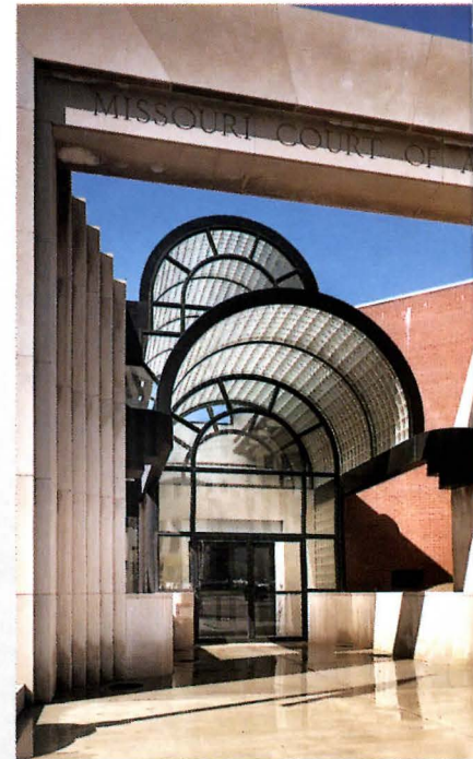
Missouri Court of Appeals, Kansas City, MO Architect: Abend Singleton Associates, Inc. DECORA® Pattern
