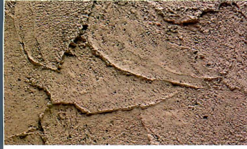
English: A thick, textured second coat is applied in varying directions in short strokes with a rounded trowel, leaving a rough, irregular pattern.
