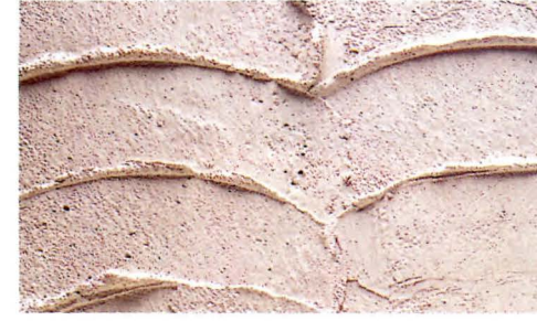
Trowel Sweep: A second coat is applied with overlapping fan-shaped strokes to form narrow, high ridges where mortar flows over the toe of the trowel.
