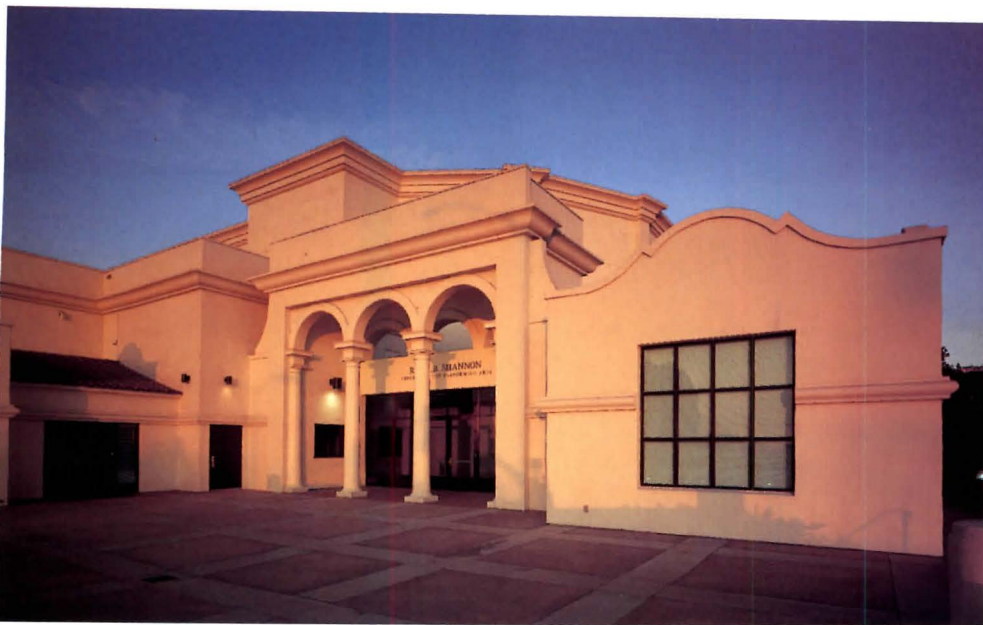
Exterior wall of Whittier College Performing Arts Center (above) by A.C. Martin and Associates of Los Angeles consists of 1-inch-thick stucco on wire mesh over gypsum
