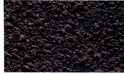
Tunnel Dash: A first dash coat produces complete coverage. When the surface has dried a day later, a second, heavy texture coat with a reduced water ratio is applied.
