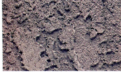
Heavy Lace: A first coat is troweled or dashed to completely cover base. Once the surface moisture dries, a second coat is troweled over it in random directions.
