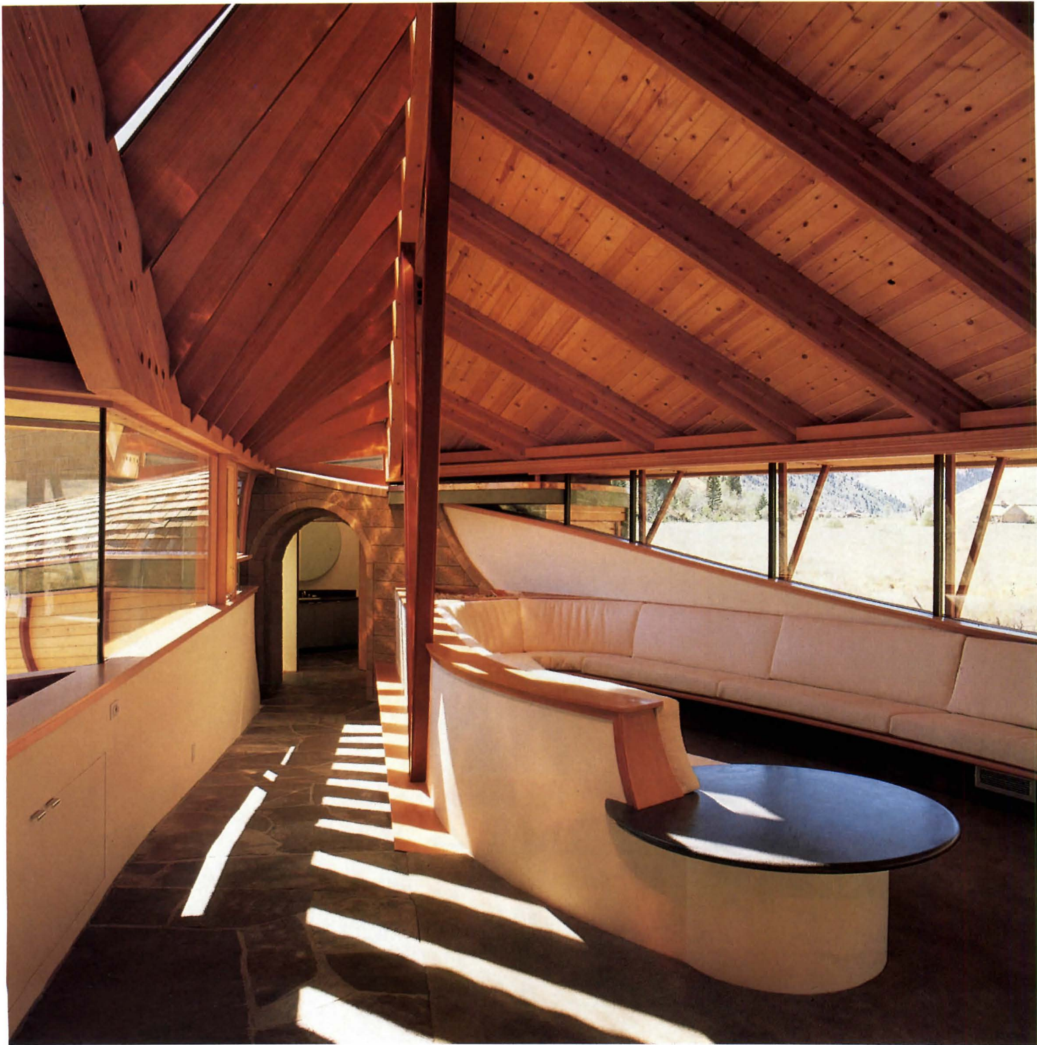
The sculptural qualities of the Whiting House are captured in the southwest corner where windows, light, and structure converge in a conversational seating area (below). Arched portion of section (facing page) shows one of two glulam beams, supported by V-braces, that define ridge shell roof.
