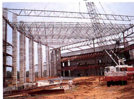
Our super long span joists easily bolt together on the job site.
