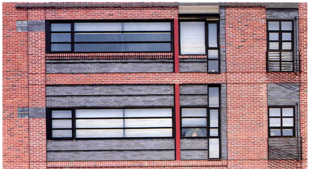
Exploded axonometric (above) depicts the thin layers of the building’s facade (below): brick, glass, and steel. Dark brick bands repeat patterns from the original building.
