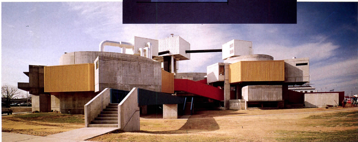
The Oklahoma City firm's renovation of John Johansen's Tinker-Toy-like assemblage (bottom) upgrades the 1970 theater's mechanical systems, energy efficiency, and site orientation. New outdoor lighting (top left), interior design elements (center left), handicapped access, and concessions areas are intended to make the building more appealing to local users while maintaining Johansen's esthetic. The project will begin construction in early 1991.
