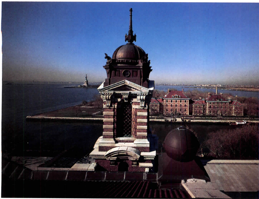
In addition to designing improvements, restoration work demands on-site presence to record existing conditions and determine what elements can be salvaged and what must be replaced. For the four towers atop the main building at Ellis Island (left), the architects decided that the wooden framework could be repaired (above), but the copper cladding would have to be replicated.
