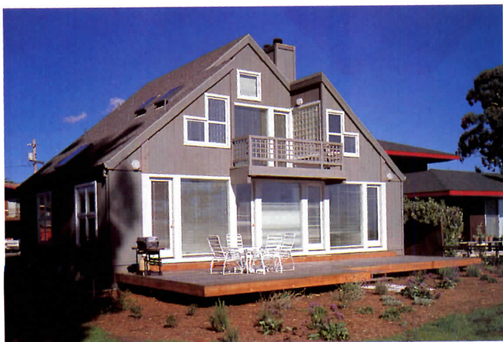
Located in Aptos, California, just 10 miles from the epicenter of the Loma Prieta earthquake, the Gaspich residence (above) survived the October 1989 disaster without a crack. One reason the 2,200-square-foot beach house performed so well, according to architect Elsbeth Newfield, was its incorporation of plywood shear walls. The exterior shear walls were designed according to Uniform Building
