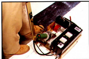
Self-propelled, hot-air welding machine fuses HyChoice seam.
