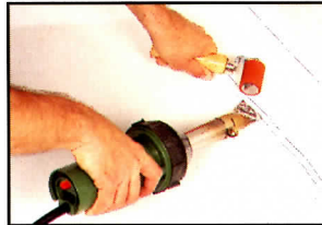
Hand-welding a field seam in a confined area.
