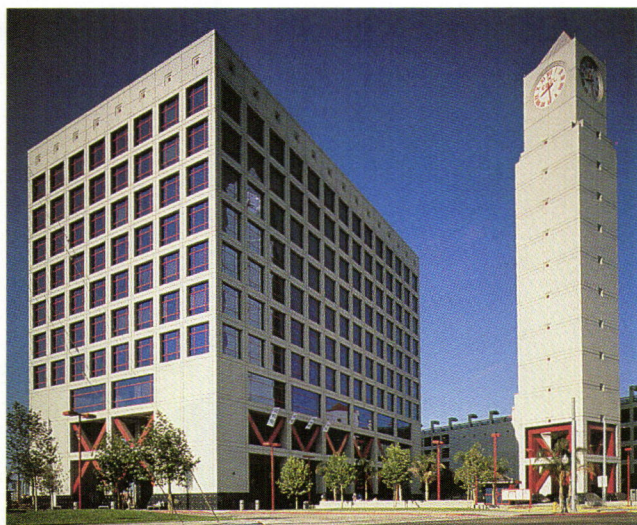
A high-rise building application rendered in a Sto EIFS (above). Craftsman trowels on the finish coat, the last step in an EIFS application (left).
