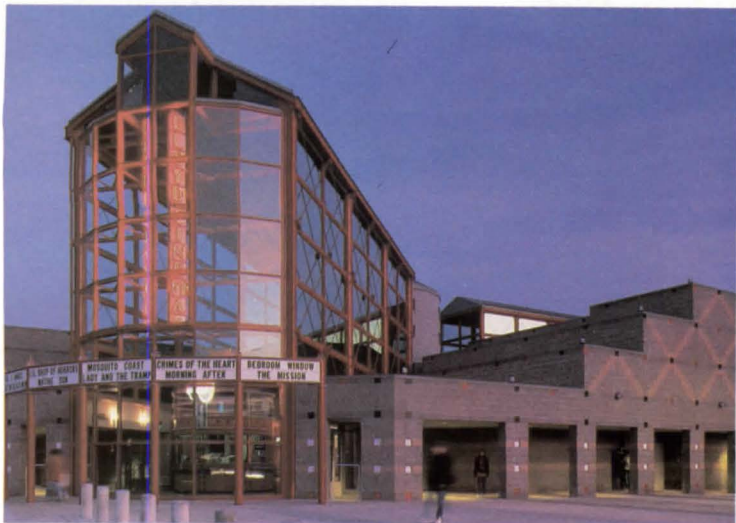
Left, the dazzling Lloyd Center Cinema. Right, the terra-cotta facade and intricate, inviting courtyard of the Institute for Advanced Biomedical Research, perhaps Portland's most striking recent building.
