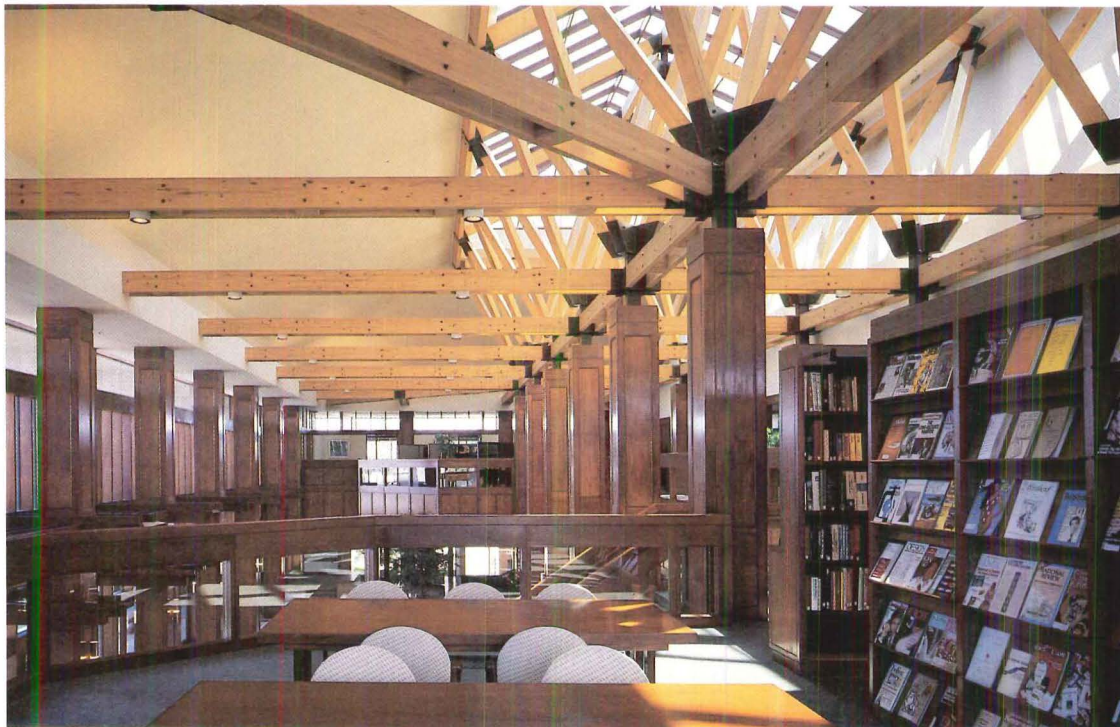
Above, main hall with central stair in distance. Mahogany columns and riggers at right in photo are rendered in cedar as they project through east wall and hover over reflecting pool, right. Left, mezzanine from library, north
