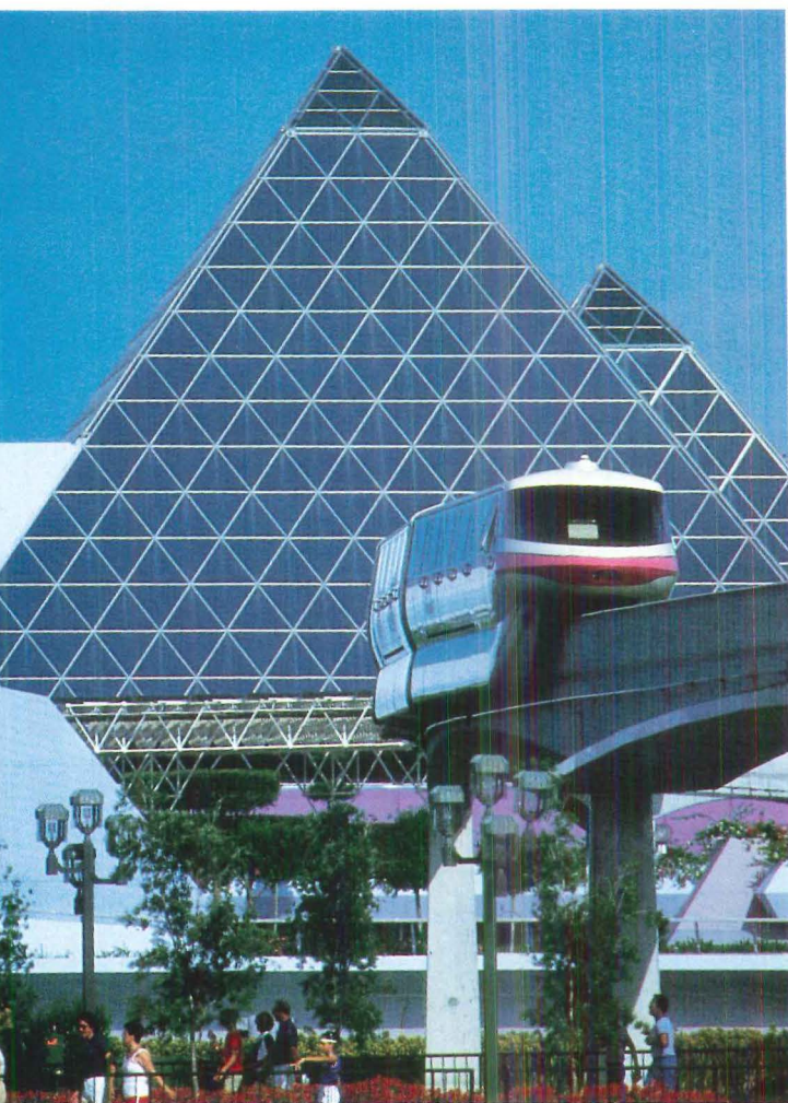
Above, the Journey into Imagination pyramids of glass as a backdrop for the Disney monorail (which runs between EPCOT Center and the Magic Kingdom). Above right, the World of Motion's stainless steel building. Right, centrally located, the Communcore's pastel-colored concrete walkways lead to a central plaza.
