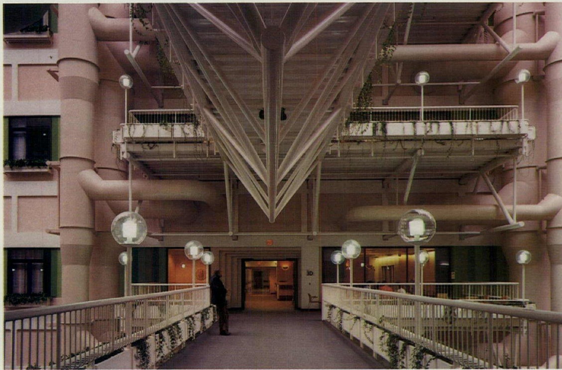
Above, bridges and elevators from northwest corner of atrium. Left, pipe trusses support bridges and balconies, and tubes thread through the structure. Right, the west leg of the atrium from the south.
