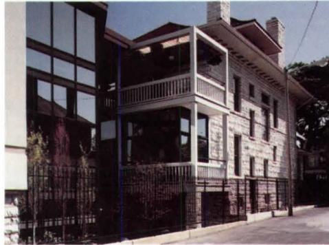
Figure 12 Stanley D. Lindsey Office Building, Nashville
