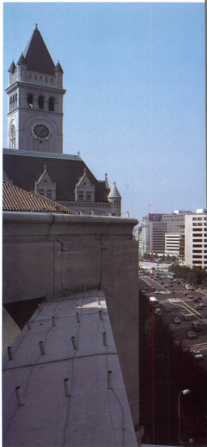
Above, Pennsylvania Avenue elevation and 10th Street facade with embedded 1909 building, seen also far right. Right, unfinished N Street elevation embedding smaller buildings.
