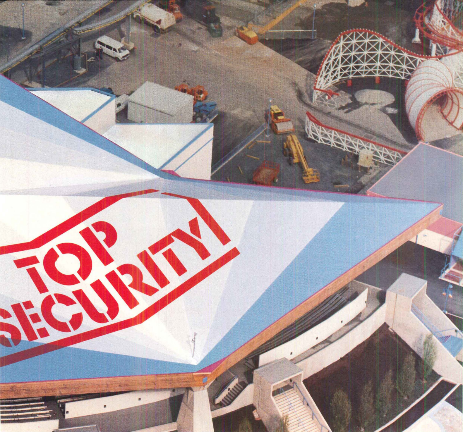
Contractor: More-Ply Roofing Roofing Manufacturer: Dunlop Construction Products, Inc., Mississauga, Ontario, Canada; Duseal Hypalon® H301 System
