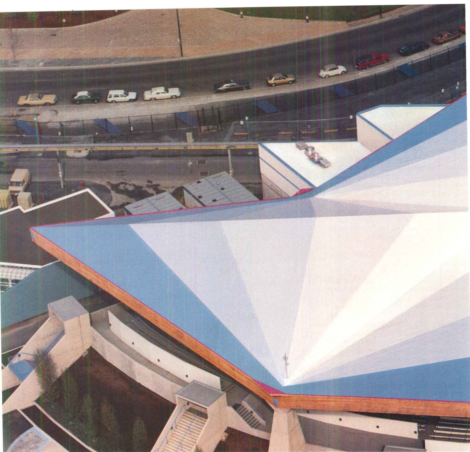
Building: Expo '86 Theater, Vancouver, Canada Architects: Aitken Smith Carter Partners; The Wade Williams Part
