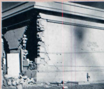
Shear forces generated by seismic ground motion, wind, and snow load are especially devastating to rigid structures. Because wood-frame design is more elastic, it dampens these stresses for higher margins of survivability.
