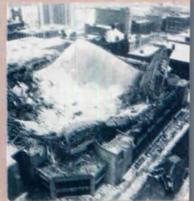
Shear forces generated by seismic ground motion, wind, and snow load are especially devastating to rigid structures. Because wood-frame design is more elastic, it dampens these stresses for higher margins of survivability.
