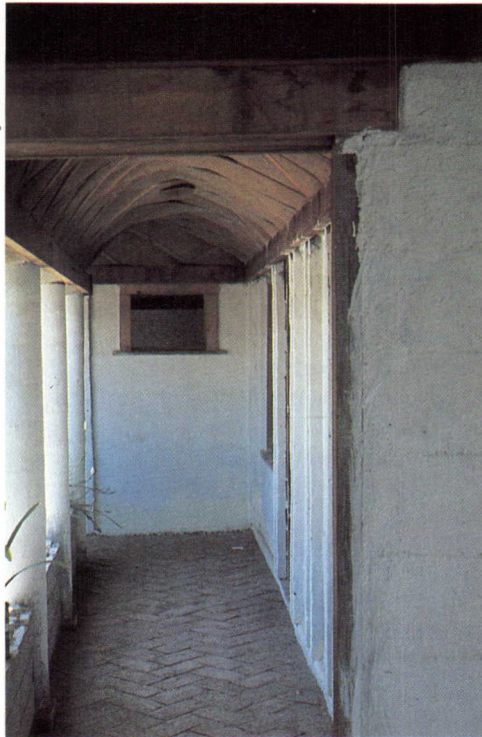
Top, courtyard side of one of five houses built during Alexander's Mexicali project; above, sunlit corridor of a Mexicali house, with burlap and basket weave vault.
