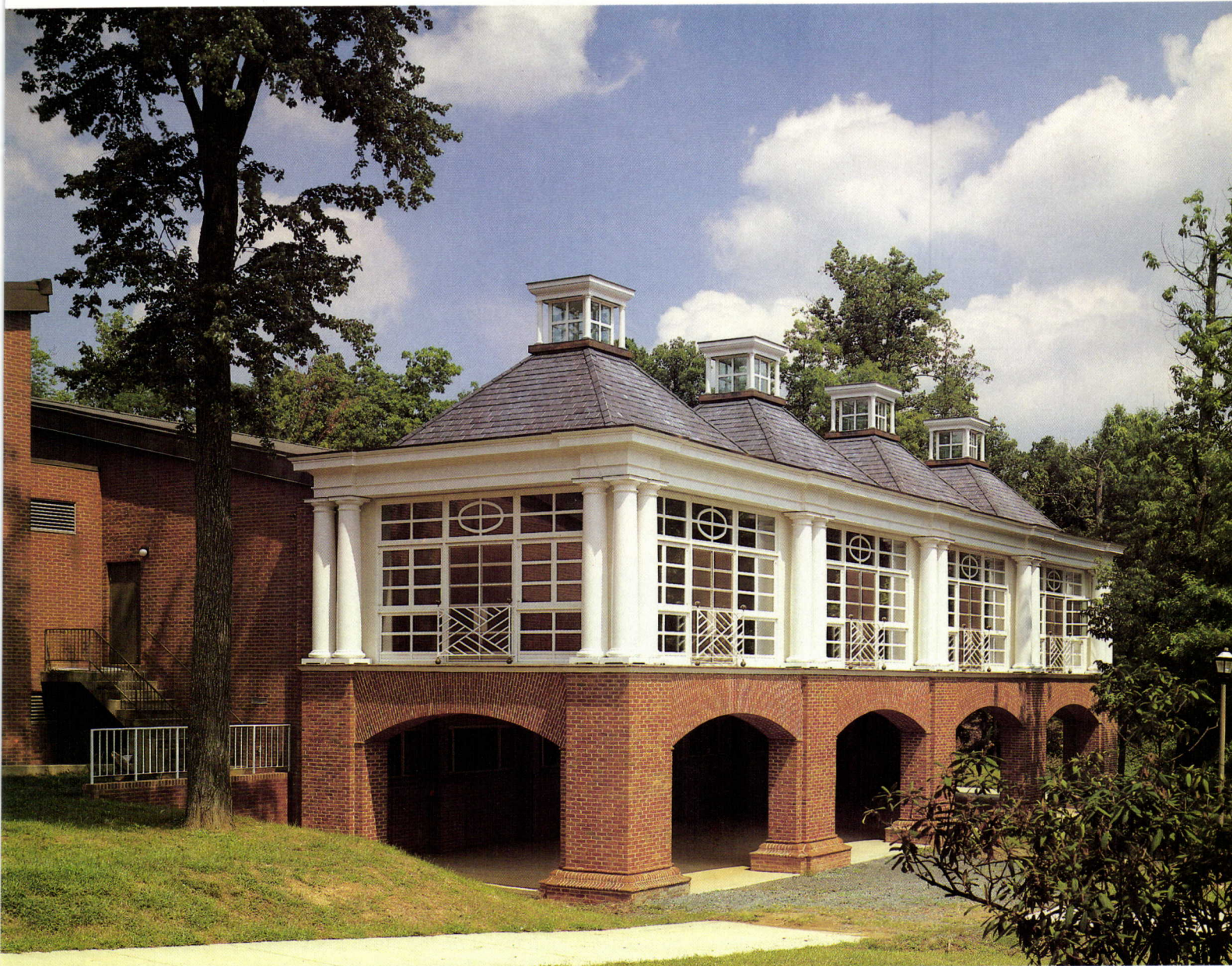
Above, quartet of hip roofs on Stern's addition to Observatory Hill Dining Hall provides light-filled room, right. Far right, new meets old.
