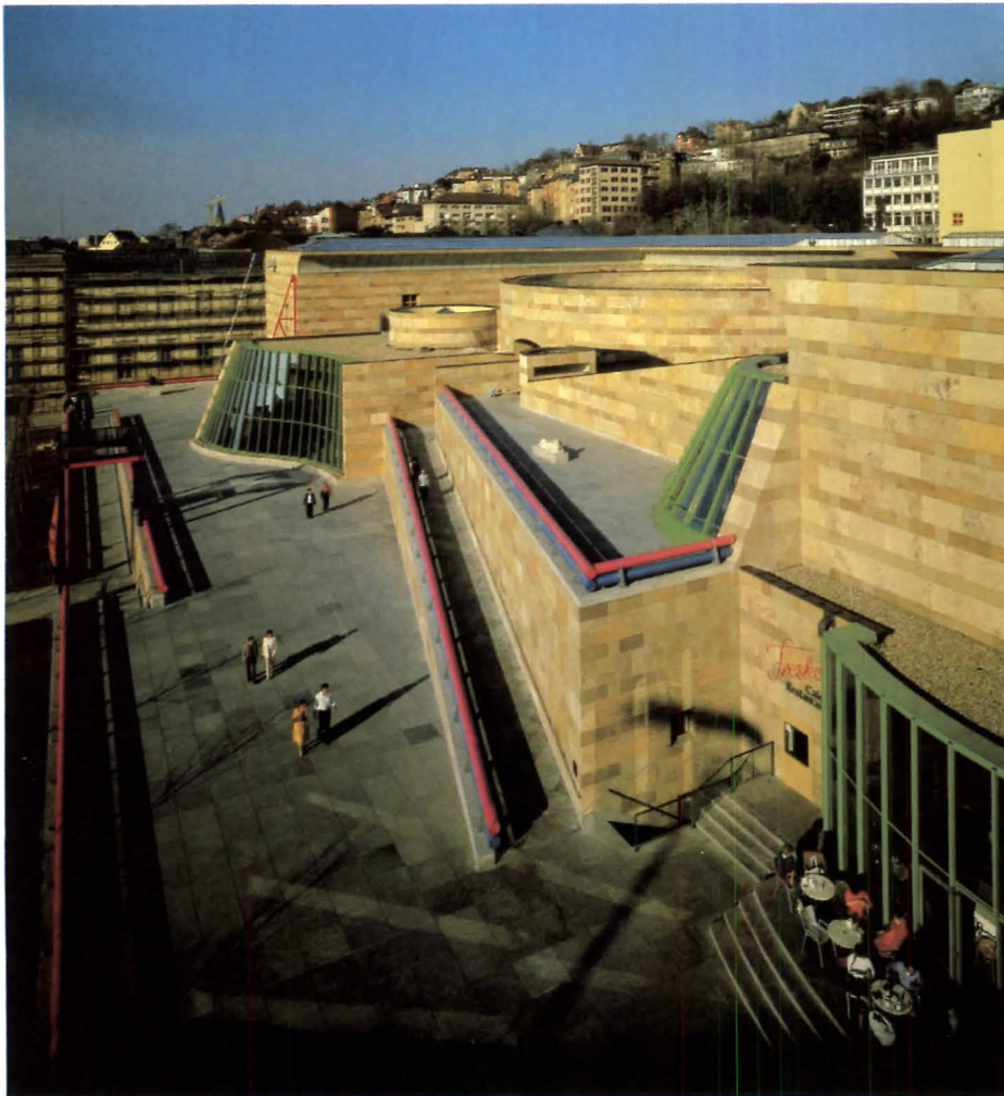
This page: left, southeast view; below, lobby. Right below, an upper level gallery; right, part of enfilade.
