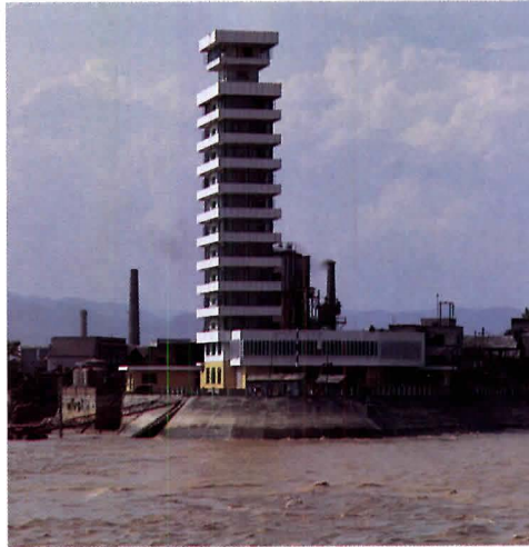
Top, Great Wall Hotel, Welton Becket Associates; above, modern office tower at Yangtse River Dam, Hubei province.
