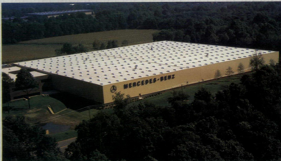
Building owner: Mercedes-Benz of North America, Inc.; General contractor: Vantage Company; Roofing contractor: Mueller Roofing Service, Inc.
