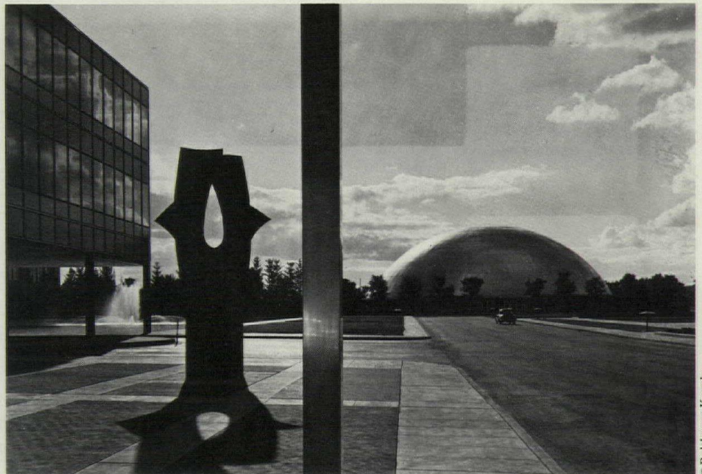
Technical Center's machine-like forms.
