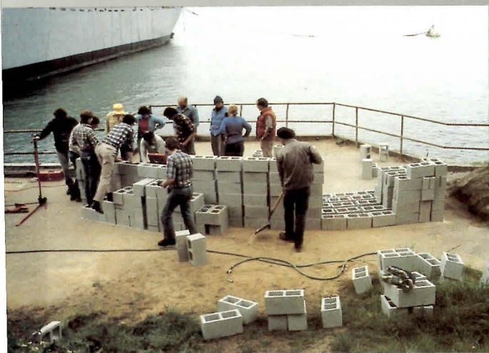
Segment of mock-up is removed for study.
