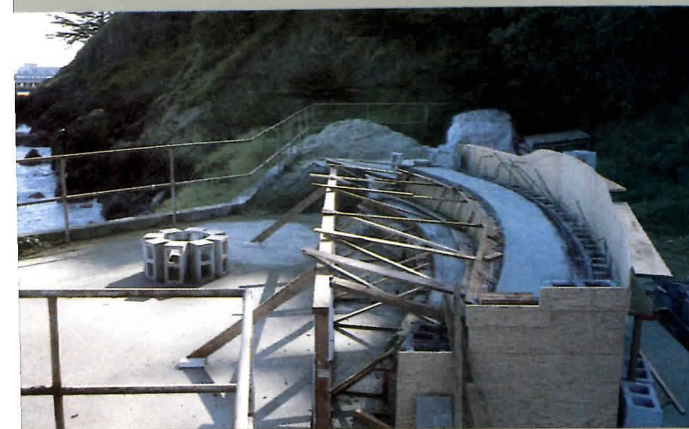
The bench takes shape after second pour.
