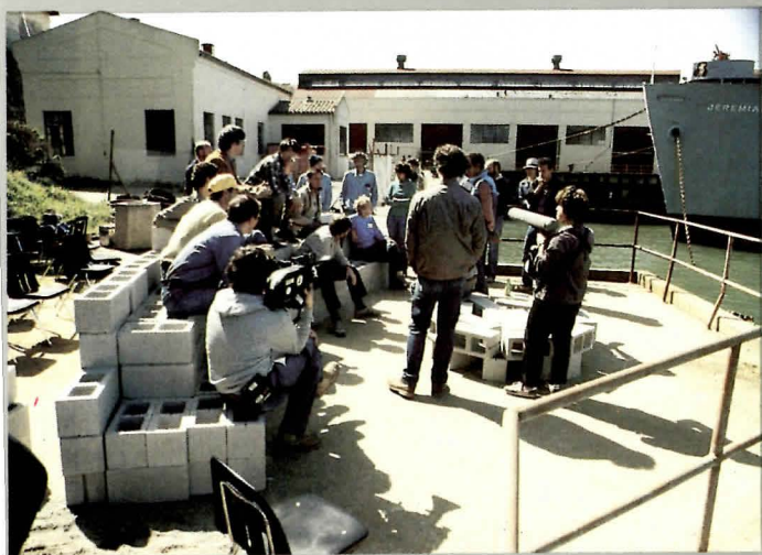
Placing the blocks in a gentle curve.
