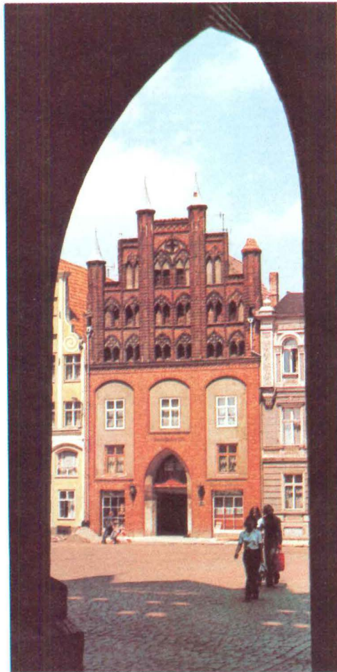
Occupying a choice place in the marketplace in Stralsund, this town house has a Gothic pilastered gable that dates from the 14th century (substructure altered in 1927-28). Its verticality allows several stories for storage of merchandise.
