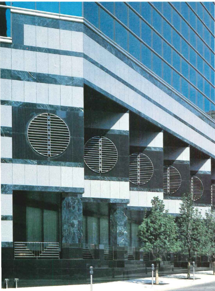
Opposite page, 333 Wacker presents rectilinear planes toward the Loop, with the circular stairs announcing the main entrance and the column and stainless steel air grilles set in marble protecting a pedestrian arcade. Left, the base consists of horizontal bands of gray granite and green marble decorated by grilles and hand railing. Above, circular stairs lead to the two-story circular main lobby.
