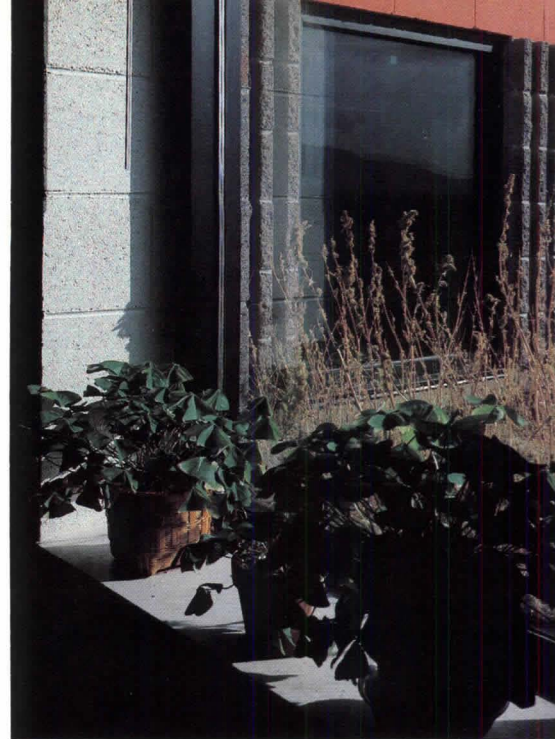
View from the interior, looking out, showing the extensive use of concrete masonry for passive solar heating and cooling and structural purposes.
