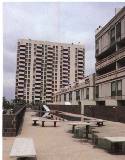
Above, Camci with Descon/Concordia in foreground, Jersey City; above right, top to bottom: TRW, Sacramento; Inland-Scholz, Indianapolis; FCE-Dillon with Pantek in foreground, Sacramento; boarded up Material Systems units, Indianapolis.
