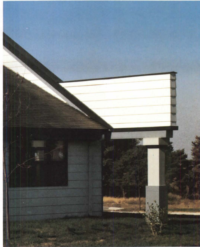
The Missouri halfway house, above and right, has a carefully worked out plan and sprightly facades that are, in effect, false fronts.
