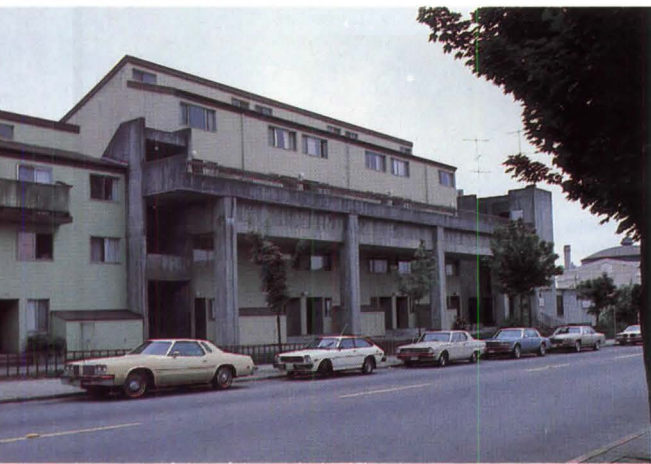
Townland system in Seattle as built, left, and a conceptual drawing of assembled units on prefabricated concrete decks.
