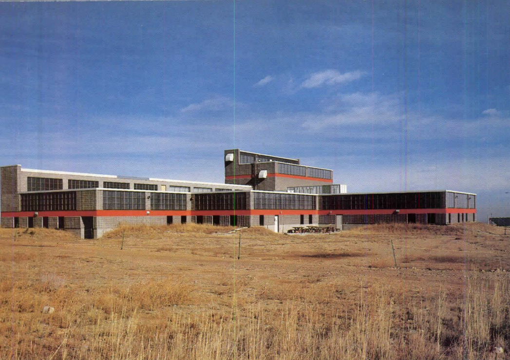
Concrete masonry Trombe walls are located behind the glazing which borders the upper portions of the building.
