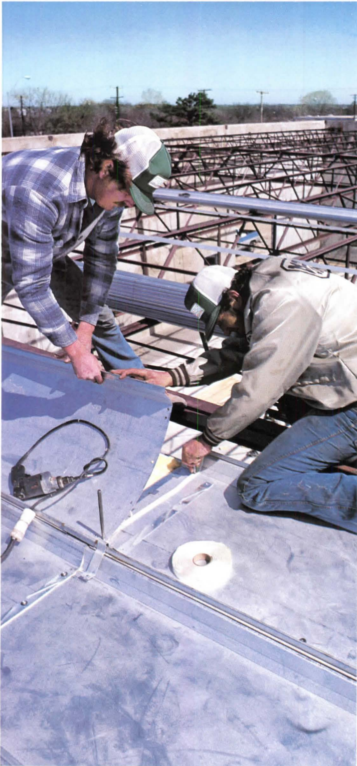
Vulcraft's unique pre-punched, pre-notched end lap assures proper installation and weathertightness.
