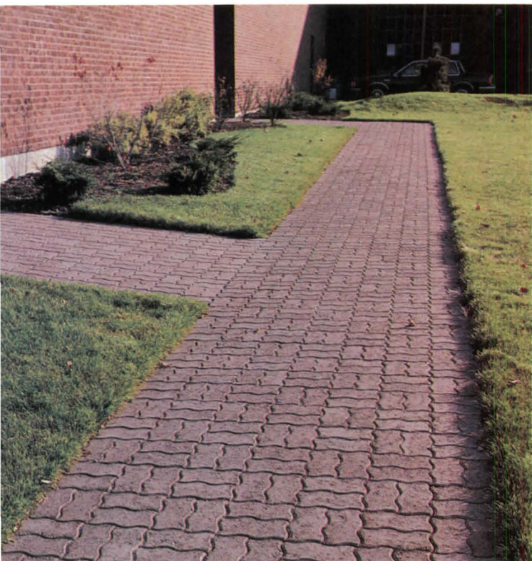
Marathon Electric Manufacturing Company, Wausau, Wisconsin. Architect/The Zimmerman Design Group.
