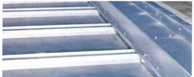
Roof-wall interface details for parapet wall.
