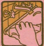
the caulk squirts out slowly. As it does, draw the spout along the tub/wall seam. When you've got the seam completely filled in with a solid line of caulk, smooth it out with a wet forefinger or a spoon handle. Let dry.
