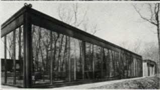
Exposed COR-TEN steel and insulated solar bronze glass are used to elegant advantage to make this 5,500-square-foot house in Lake Forest, III., (above) mirror its handsome wooded setting. Architect: Clarence Krusinski & Associates. Merit.
