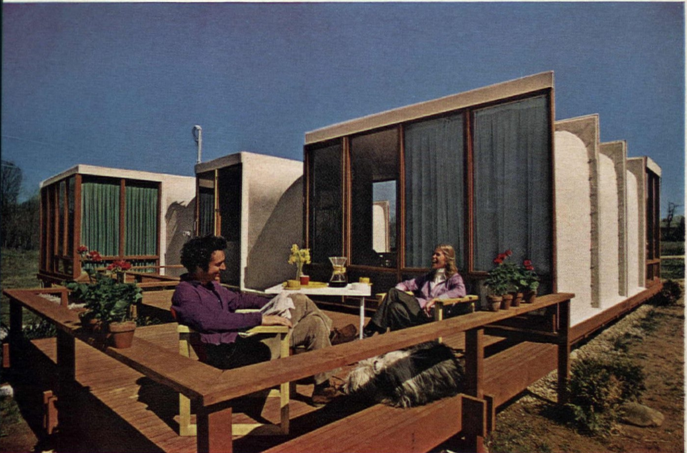
Designer Mark Hildebrand (above) relaxes on the deck with classmate Mazie Cox from the Yale School of Art and Architecture. Ribbed exterior clearly shows how the modules are bolted together.
