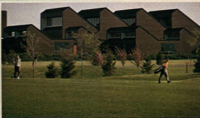
Edward Larrabee Barnes was architect for the W. D. Richards Elementary School (above). Overlooking a public par-three golf course, the school is a community focal point.
