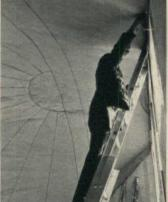
Foam is applied by means of a spray gun. The urethane mixture, combining a resin and an activator, can be varied to
