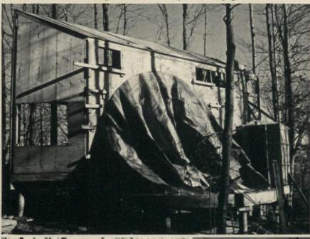
The foaming process begins with a bag, in this case one of bonded paper and polypropylene that arrived on the site as a roll to be cut into sections and sewed to required size.
