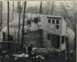
Inflated by a standard office fan, the bag is coated with Canadian Industries' 268 Series urethane foam. A quick, cost-cutting process, foaming of both domes will be completed in a day.
