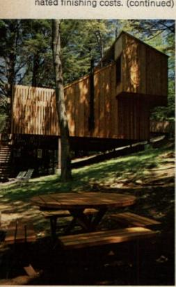
Supporting piers (above) are outside extensions of interior columns. Louvers on deck provide cross ventilation.
