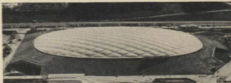
The U.S. Pavilion at Expo 70, with the largest clear span, air-supported roof ever, will house the architectural exhibit previewed on page 39 and other exhibits on the moon landings, on U.S. sport and art. It was designed by Davis, Brody, Chermayeff, Geismar, deHarak Associates.
