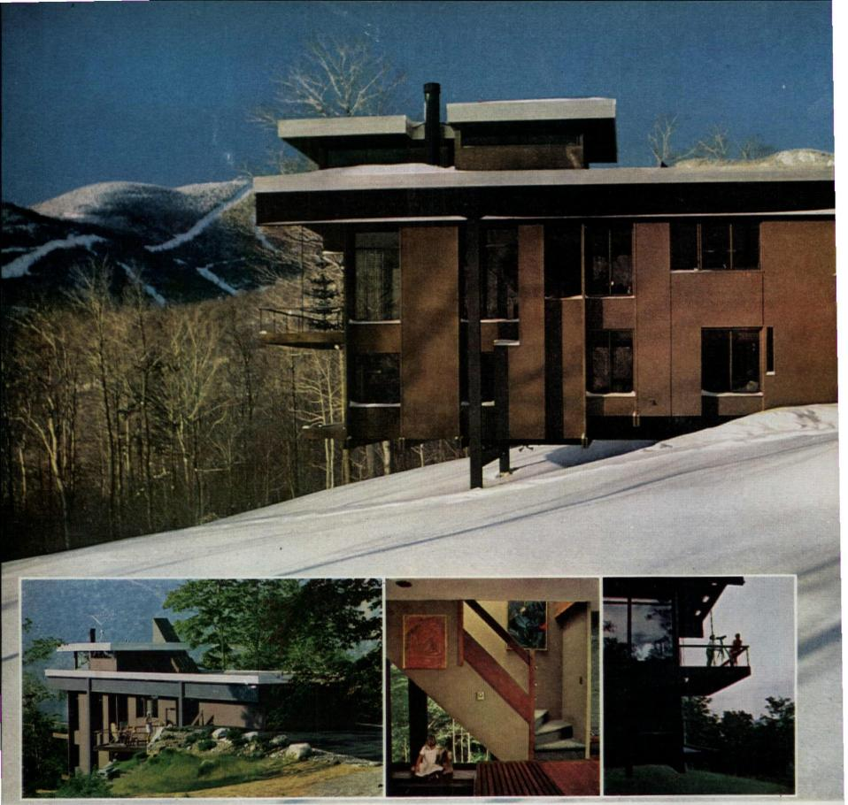
Exposed steel framework of Zimmerman house provides main support from above instead of underneath. "Cupola" on roof is master bedroom, with adjoining sun deck. Attached garage is seen in the foreground. Unusual siding was used on stairway as well as on exterior of the house. It was made by saw-cutting narrow-spaced grooves into common tempered hardboard siding, then applying three coats of paint.
