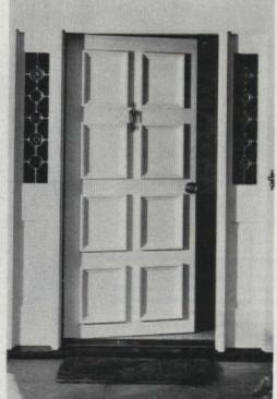
Here the moldings were mitered, then fastened to the door in pictureframe pattern that gives an effect similar to that of traditional panel doors. Each molding actually consists of two narrow moldings glued together before mitering. This trick is often used to vary stock patterns and sizes, or when a wide, intricate molding is required.
