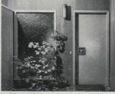
Besides merely dressing up the door, eight vertical strips of molding make this door more consistent with the vertically slatted privacy screen to its left. In addition, they create eye-catching shadow lines that make the door stand out visually from the plain walls. Strips are applied with brads and waterproof glue.
