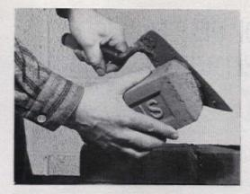
"Butter" the end of each brick before sliding it in. Slice the mortar on end, then shape it on four sides to a peak, like a pyramid. This helps make it stick while you lay it.
