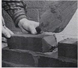
Lay each brick an inch or so from the one preceding it. Press down slightly, and forward. With practice, you will soon be able to apply mortar for several bricks at one time.
