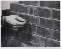
Treatment of mortar joints is very important in weatherproof masonry. Tightest joint is made with flat striking tool or rounded "sled runner" used with troweling stroke. Hold tool at angle shown to achieve the best weather-proof joint.
