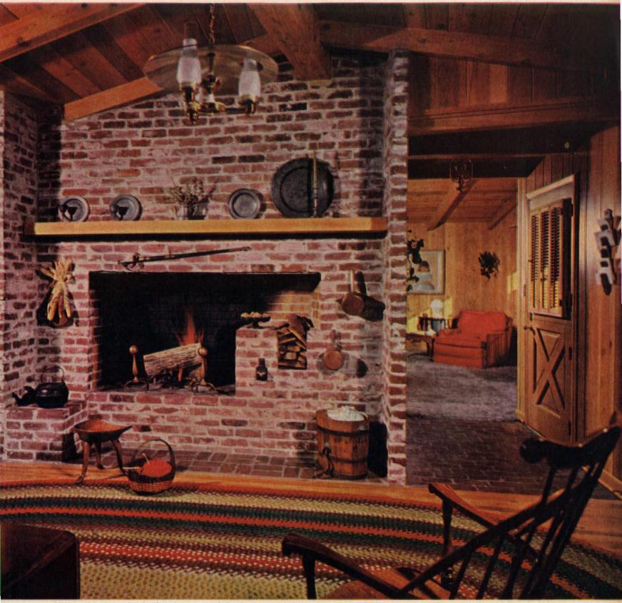
Giant fireplace in the keeping room of the Butler home is double, opening into both this room and the living room. It's built of used brick, as are the floor and wall of the front entry
