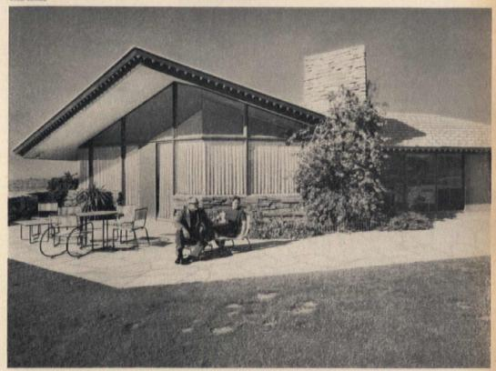
Triangular theme of house is apparent in roof pitch, patio design, and triangular metal dentils used as ornamentation on the overhang. The kitchen wing is at right. Roof shingles of lightweight concrete provide excellent insulation against the brilliant Arizona sun.
