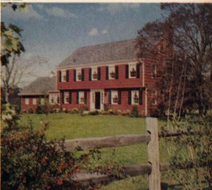
This handsome colonial house with split-cedar shake siding, slate shingle roof, and chimney made of used brick is perfect in proportioned detail. It was designed and built by Walter Uhl.
