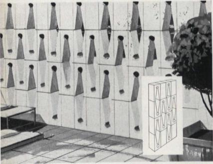
Keyhole-shaped lintel blocks, placed foot to foot, form a diamond pattern. For alternation of the diamonds, double corner blocks are spaced between the lintel blocks on the bottom and topcourses.
