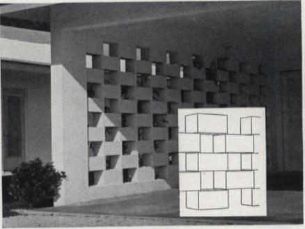
Double corner blocks stand here in a pattern as old as children's blocks, and just as satisfying. Excellent for a windbreak, or for the end wall in a carport. Support must be provided for end rows.
