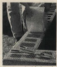
Use wire mesh reinforcing on the next-to-top course on all walls, and along every fourth course on high walls. Use vertical reinforcing rods if stronger support is required.
