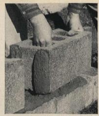
To lay succeeding blocks, stand them on end and "butter" inside and outside corners. Tap with the trowel to seat the mortar, keeping it from falling off in transit.
