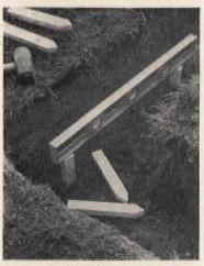
To insure that the footing is even, drive stakes into the bottom of the trench; use a level to make sure the tops of the stakes are all the same height.
