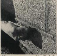
Mortar courses must be "tooled" to make them firm and water-resistant. This is true even when the joints are to be kept flush. The tool shown is the simplest; there are also tools to produce a v or concave joint.
