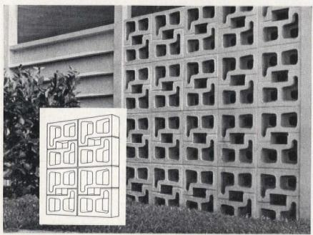
Corner blocks, like the chimney blocks shown at left, present an intricate design when placed on their sides. Stacked corner-up, corner-down, the resulting grille seems modeled and hand-crafted.
