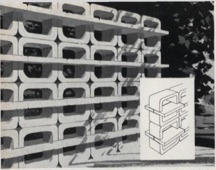
Half-column blocks clamp pairs of flat patio blocks for a shelved, horizontal effect. Less for screening a view than providing a backdrop, this fence gives free ventilation, needs a 16" width allotment.
