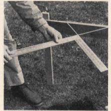
Use "batter boards," cord, and a framing square to lay out the trench for the footing. Corners at ends of wall must square with each other. Nails in the crosspieces that hold the cord should be at the precise line of the wall.
