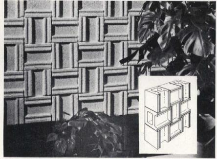
Half blocks with stretcher ends describe a strong basket-weave pattern. The simple alternating of the blocks, vertically, then horizontally, gives a light look to an otherwise heavy, solid wall.
