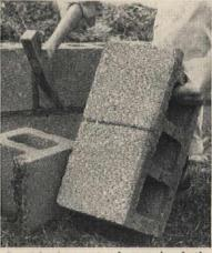
Cut blocks to size by scoring both faces with a cold chisel. Tap gently, slowly pulverizing along the line. When the line is scored, a sharp rap will break the block.
