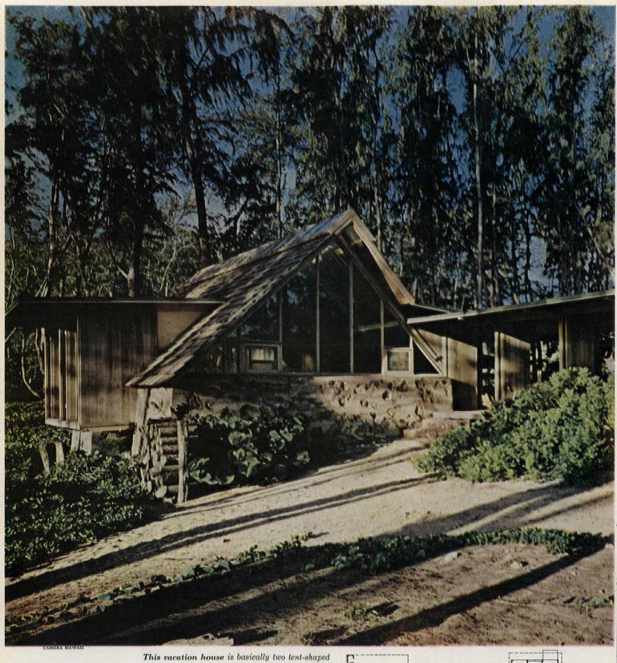
This vacation house is basically two tent-shaped structures, commonly called "A-frames," connected by a covered passageway or lanai.
