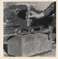
The first block is embedded in mortar and made absolutely straight and level. The blocks can be moved by applying pressure and tapping gently on the top or face. Use plenty of mortar so that the block can be forced down; then scoop off excess mortar from the joint.
