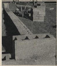
A tight drawstring is essential to keep the blocks in a straight line, Lay one block at each corner, then stretch the string, check with a level, and lay others to it.
