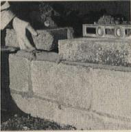
Cap the top of a garden or retaining wall with a 4" solid block laid flat. If the wall is to serve as the foundation for subsequent construction, fill cores of the top course with mortar, troweled smooth; sink anchor bolts in the core filling.
