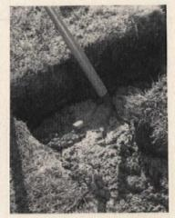
Pour concrete into the trench, allowing it to just barely cover the tops of all the stakes. Semiliquid nature of concrete makes this easy. Leave stakes in.
