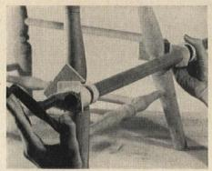
Bar clamp is well adapted for the widespread job. Buy clamp devices at hardware store, then use any pipe length necessary to fit the job.
