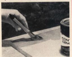
Contact cement is most often used for applying plastic sheet material to counter and table tops. Coat both the surfaces to be joined.
