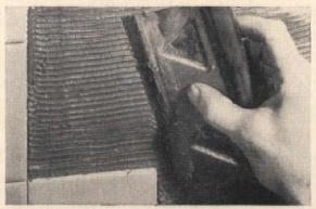
**Toothed spreader** is the usual method for applying mastics for plastic or ceramic tile, wood-block flooring, and some laminations. Spreader leaves the proper amount of mastic on the supporting surface.
