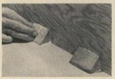
Hardwood blocks are often used to strengthen a corner. They are glued into place with a sliding motion without clamps, nails, or screws.
