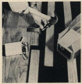
A SPECIAL NAILING PLATE (rent or buy one from your lumber dealer) protects the flooring from hammer blows, directs nails at proper angle, speeds installation.
