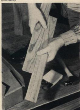
NEW FLOORING HAS TONGUES AND GROOVES on edges and ends. Lengths range from 10" to 8'. The first "course" of strips laid across the room should be at right angles to the old flooring. Also apply strips parallel to starting wall, ½" out.
