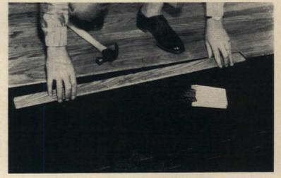
NAIL EACH COURSE FROM WALL TO WALL before starting another. Drive nails at 6" intervals and within 4" of the end of each strip. For best appearance, space end joints 6" to 8" apart.
