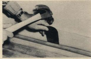
pry off shoe molding on baseboard with a piece of thin metal. If floor boards are loose or squeak, nail them tight with 6d flooring nails; countersink nail heads. If old floor surface is uneven, rough-sand it smooth.
