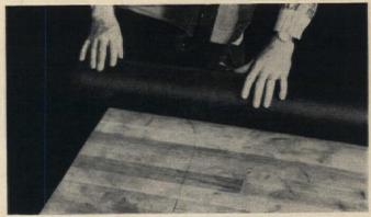
LAY 15-LB. ASPHALT BUILDING PAPER at right angles to the old flooring underneath, overlapping edges 4 inches. This will protect the new floor from dust and moisture. (continued)
